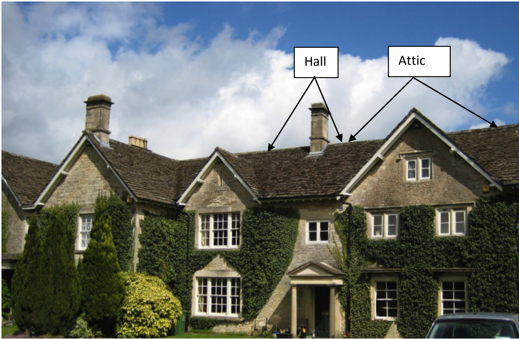
Figure 3: General view of west (south-west) elevation of The Old Rectory showing locations of the open hall and attic roof
