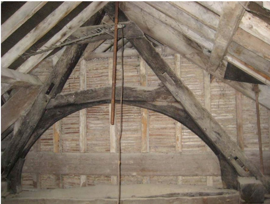
Figure 4: South face of open hall truss A
