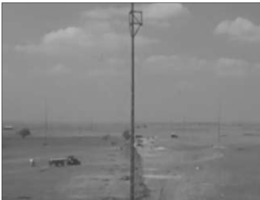
Figure 15: Image looking along the MUSA during construction. In the distance, one can see the faint outline of the telegraph poles used to construct the rhombic antennae (still from Jennings 1938 © Royal Mail Group Ltd 2011, courtesy of The British Postal Museum & Archive).
