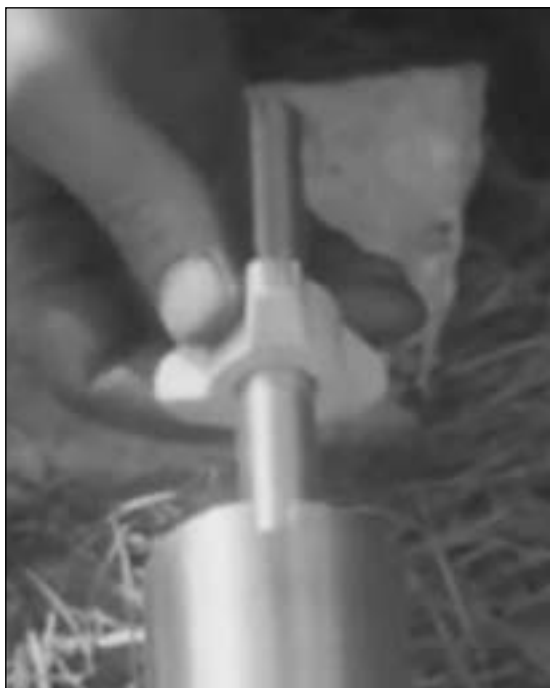
Figure 17: Three-legged spacing insulator (still from Jennings 1938 © Royal Mail Group Ltd 2011, courtesy of The British Postal Museum & Archive).
