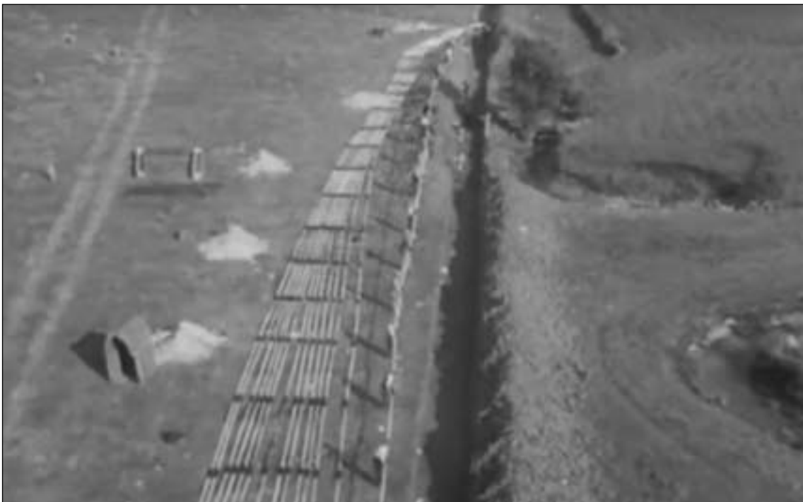
Figure 12: Laying the feeder tubes (still from Jennings 1938 © Royal Mail Group Ltd 2011, courtesy of The British Postal Museum & Archive).
