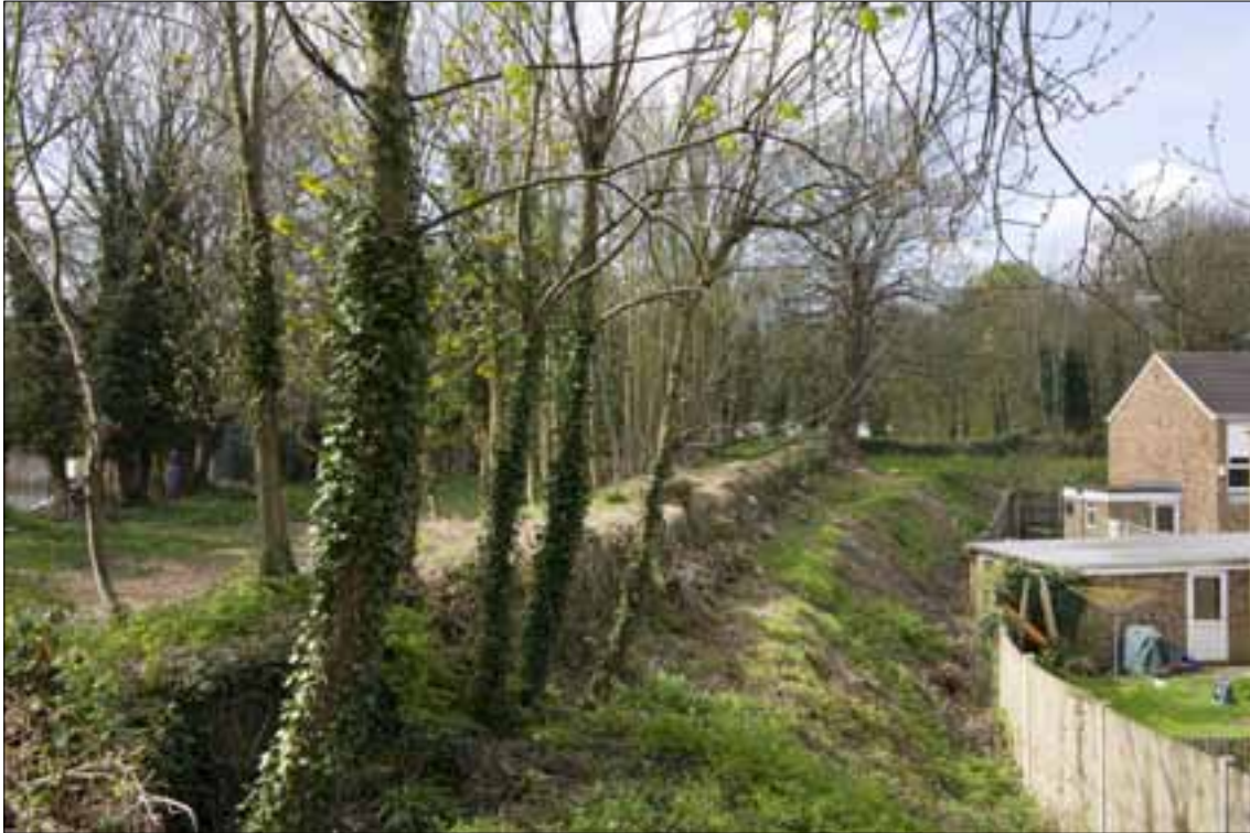
Figure 25 - Looking southwest from the salient along the south face (© English Heritage DPI 19295 Steve Cole)
