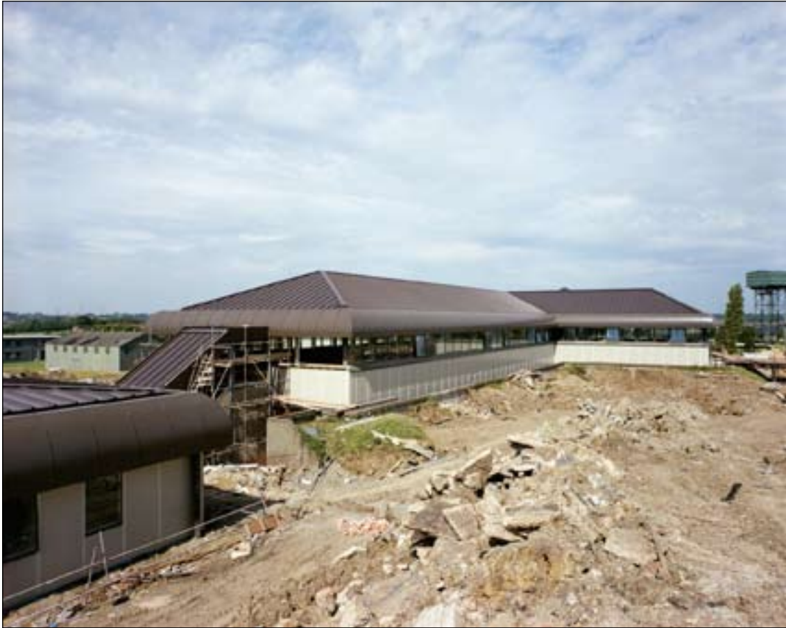
Figure 30: Extension to main Technical Building (PIG 28793/003 © Crown copyright. NMR).
