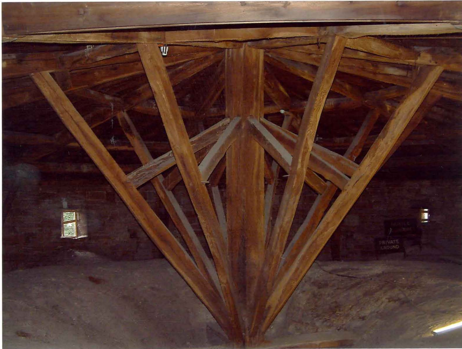
Figure 3: Worcester Cathedral, Chapter House roof (provided by English Heritage)
