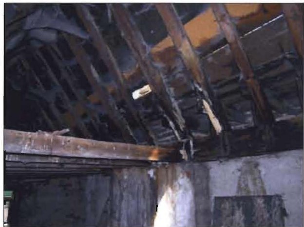
Figure 6. Detail of front roof. Pete Smith 5/10/2006
