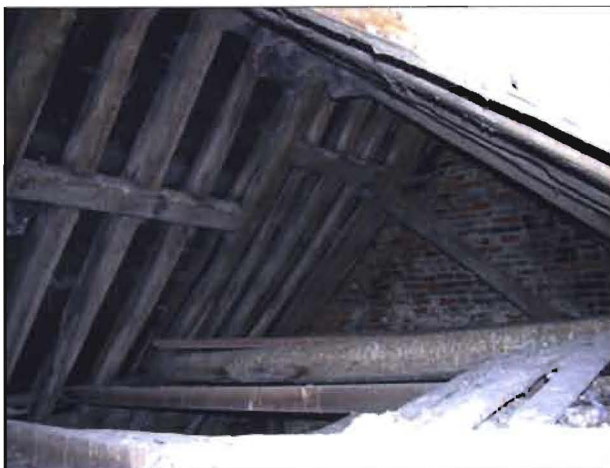
Figure 7. Interior of rear roof. Pete Smith 5/10/2006
