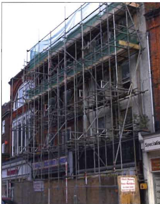
Figure 1. The main north-west front, now covered in scaffolding. Pete Smith 5/10/2006
