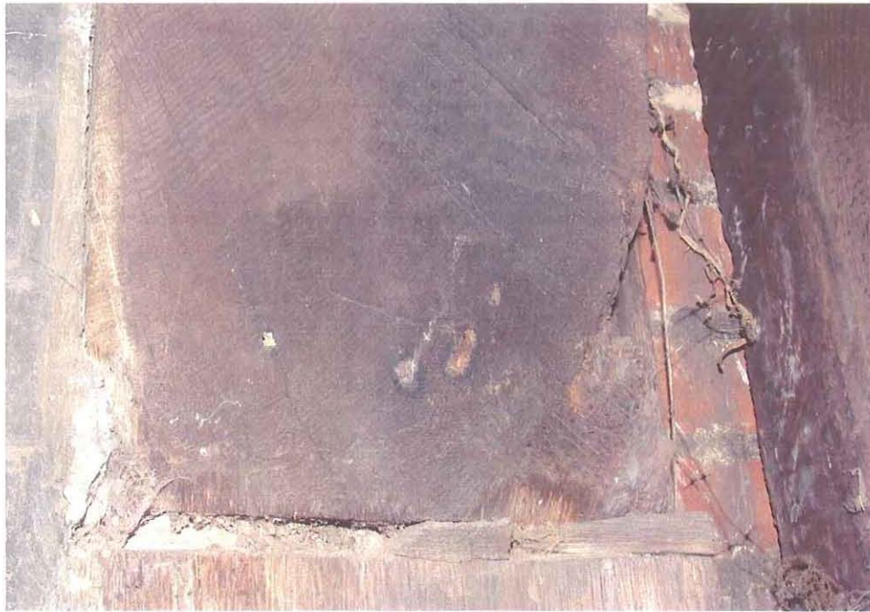
Figure 6: Photograph of the doorhead (FPG06) with complete sapwood
