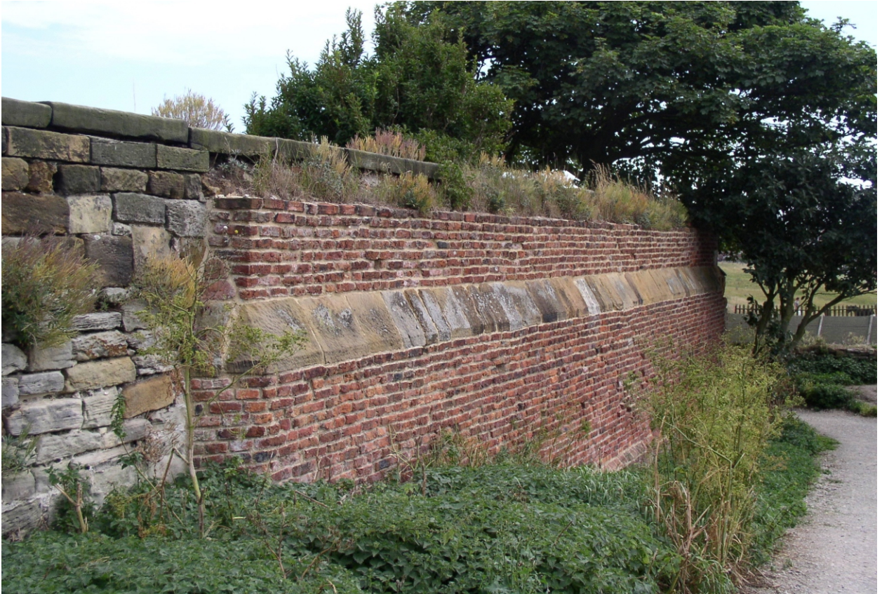
Plate 3. Area H/J West wall of Parlour Yard, junction of brick and stone, possible terrace edge
