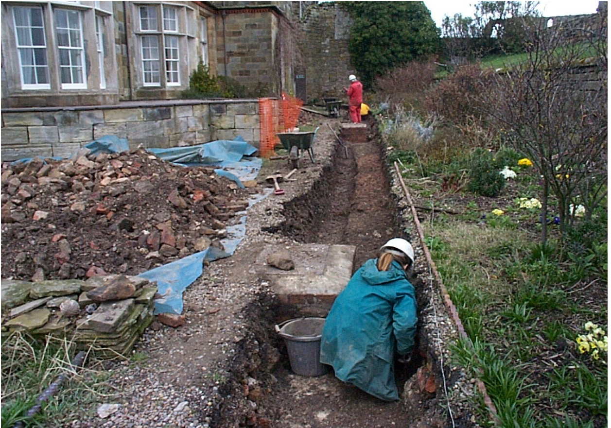
Plate 4. Site Subdivision H24, constrained working conditions, facing north
