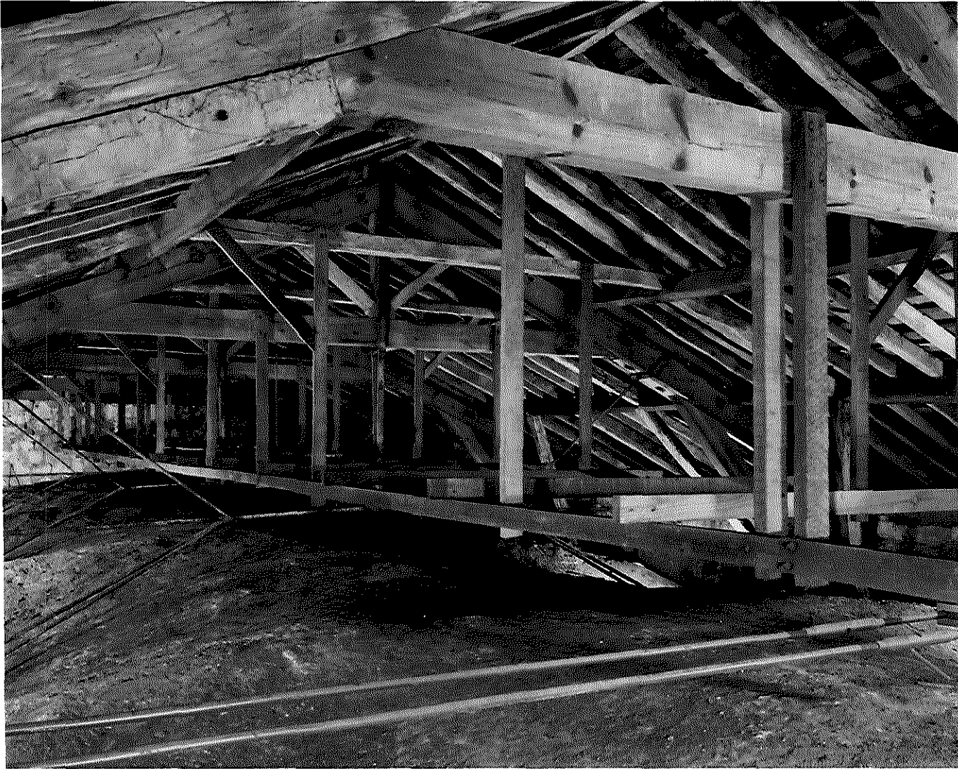
Figure 4: Photograph of the Lady Chapel roof showing the modern softwood trusses. (© Crown copyright. NMR. BB88/5843)
