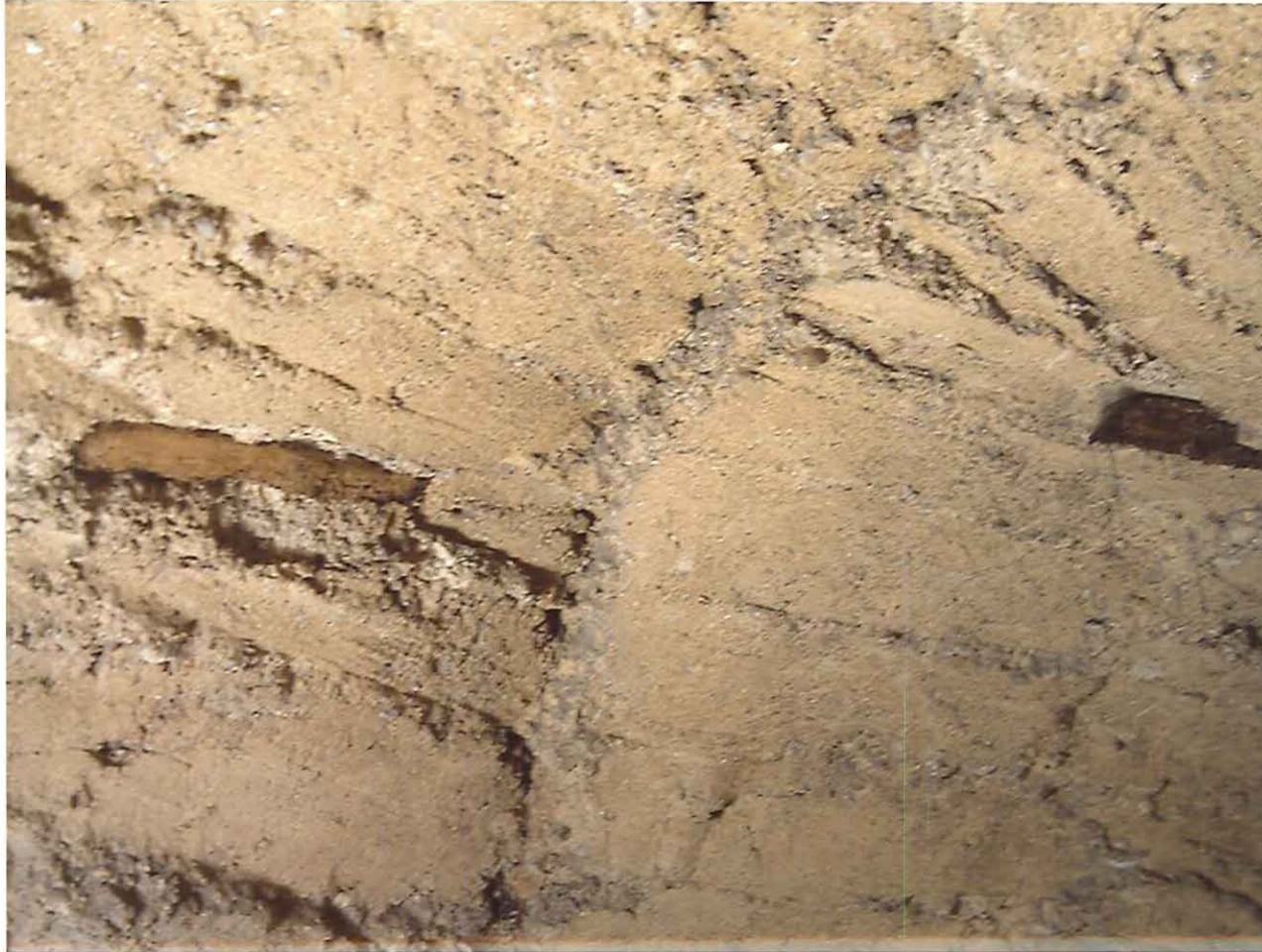
Figure 28: Photograph showing the remains of two shuttering boards (photo Dr Peter Marshall)
