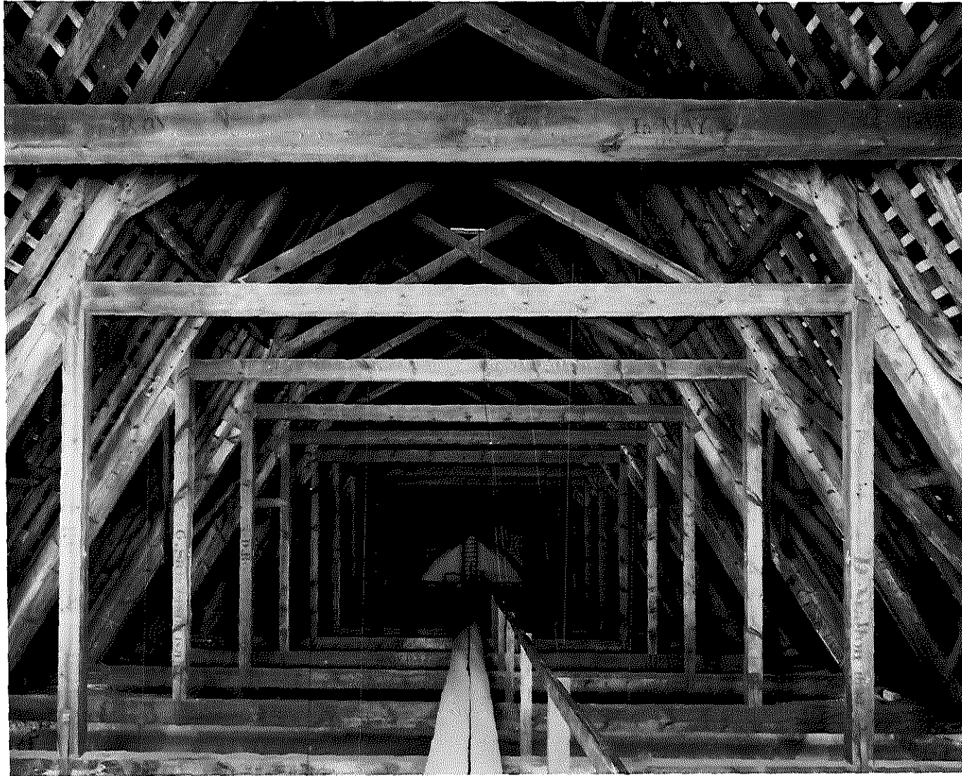
Figure 7: Photograph of the Presbytery Roof. (© Crown copyright. NMR. BB98/17656)
