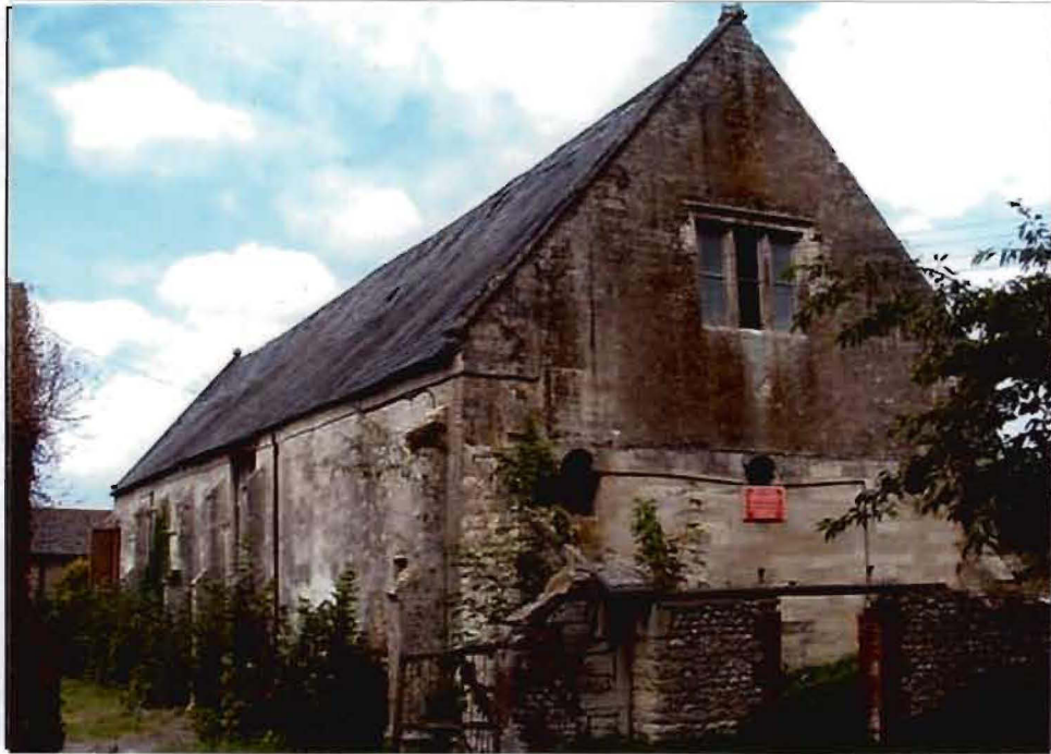
Figure 2: Exterior view of the Riding House from the south east, looking north west
