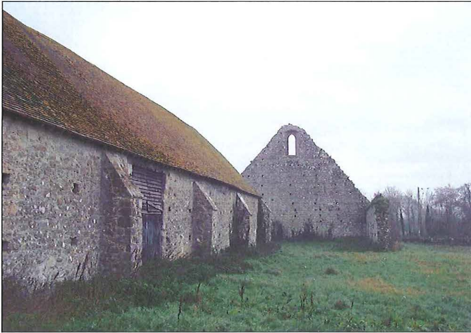
Figure 2: View of the south wall of the barn, looking east, showing its position within the remains of a once much larger barn, photograph M Bridge
