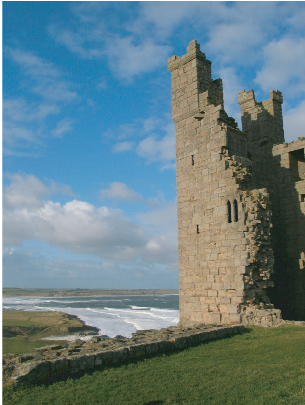
Figure 20. Lilburn Tower, seen from the south-east
