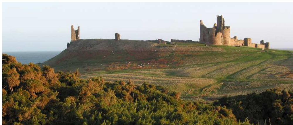
Figure 2. General view of Dunstanburgh from the west
