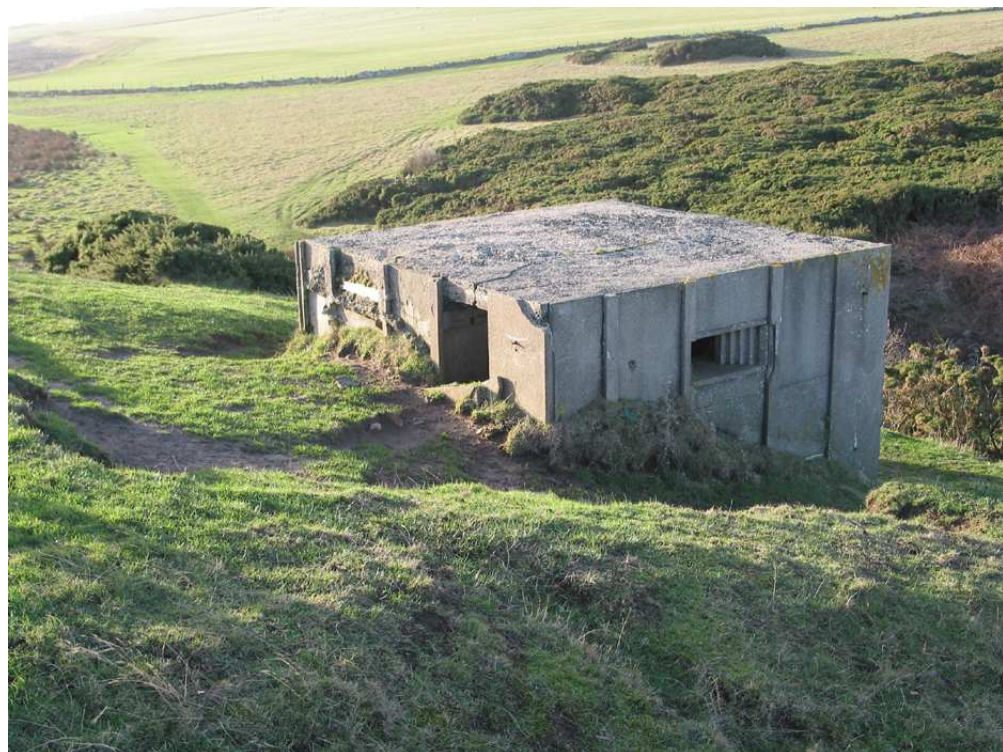
Figure 40. The pillbox, seen from the north-east
