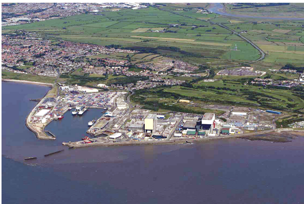
Figure 13 Heysham, Lancashire, here the power stations were built on reclaimed land, the Irish Sea providing a plentiful supply of cooling water © English Heritage NMR 20319-008
