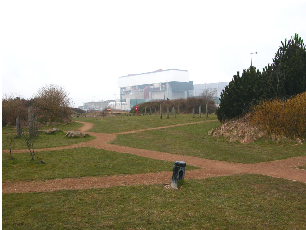
Figure 20 Heysham, Lancashire, the power station viewed from the nature reserve © English Heritage
