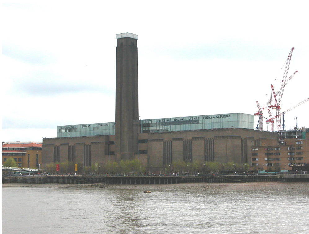
Figure 16 London, Bankside power station, now Tate Modern © English Heritage
