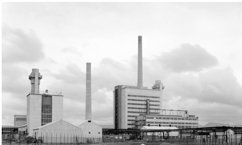
Figure 6 Windscale, Cumbria, 1954, the Windscale Piles and the ten-storey reprocessing plant used to extract plutonium, rising from which is a single tall ventilation stack © Crown copyright. NMR G5158-1
