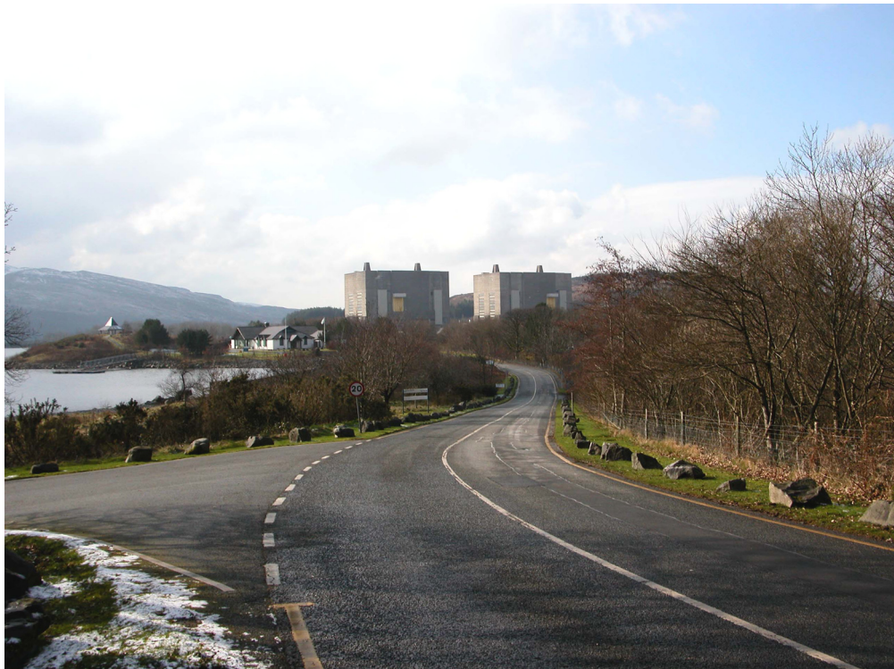
Figure 18 Trawsfynydd, Gwynedd, the visitor centre is to the left overlooking the lake, the reactor buildings were designed by Sir Basil Spence © English Heritage
