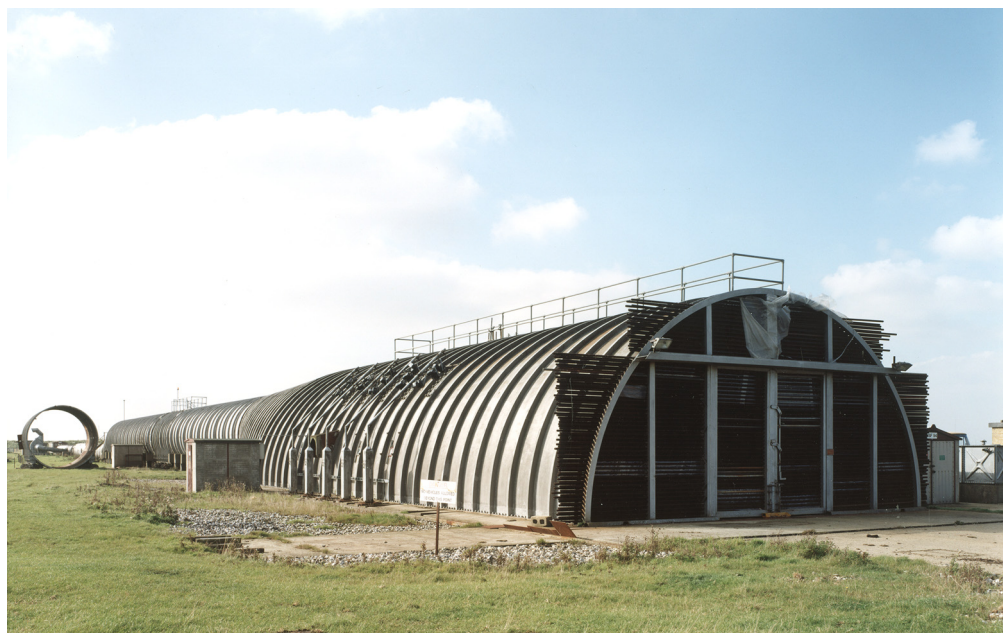
Figure 4 Foulness, Essex, air blast tunnel used in the simulation of blast waves © English Heritage BB99/15990
