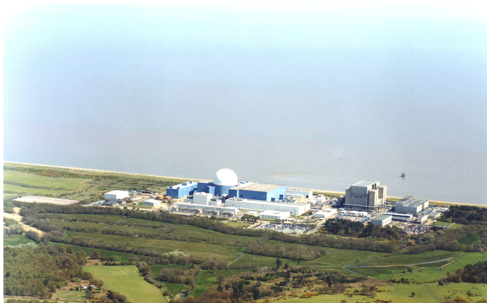
Figure 27 Sizewell, Suffolk, to the right is the 1960s Magnox station Sizewell A and to the left the is the 1200 MWE Pressurised Water Reactor © English Heritage NMR 23495/12
