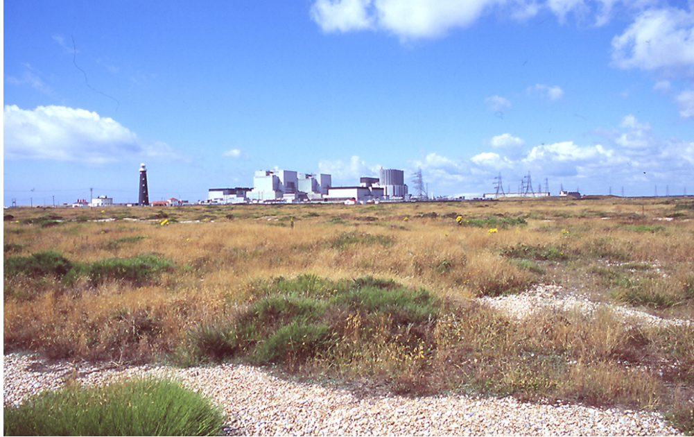
Figure 14 Dungeness, Kent, the power station in its landscape © W D Cocroft
