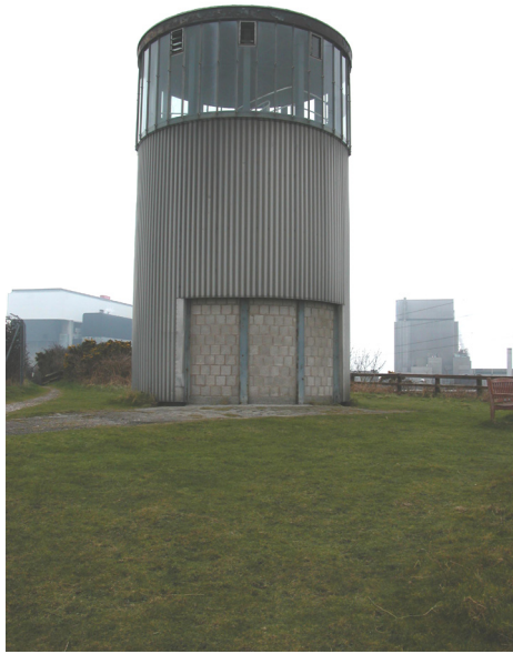
Figure 17 Heysham, Lancashire, observation tower, its entrance was bricked up after the 2001 terrorist attacks on New York © English Heritage
