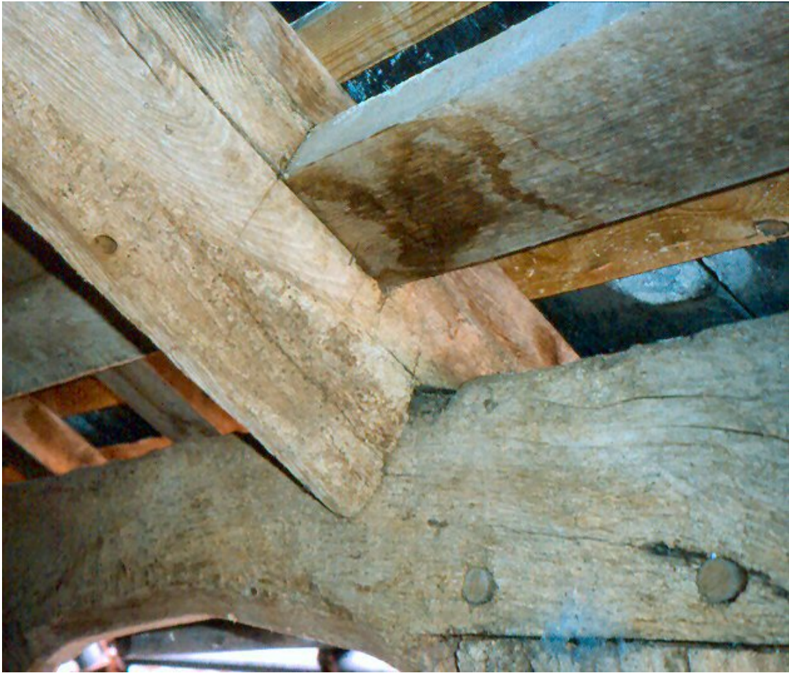
Figure 8 Detail of a shore-type truss in the gallery (photograph C Groves)
