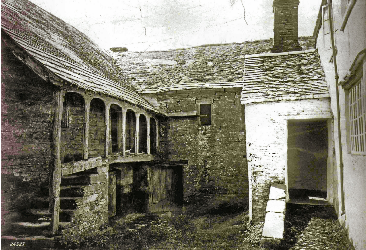
Figure 6 The stone steps and gallery leading to the upper floor of the south and west ranges (photograph reproduced by permission of English Heritage, NMR)
