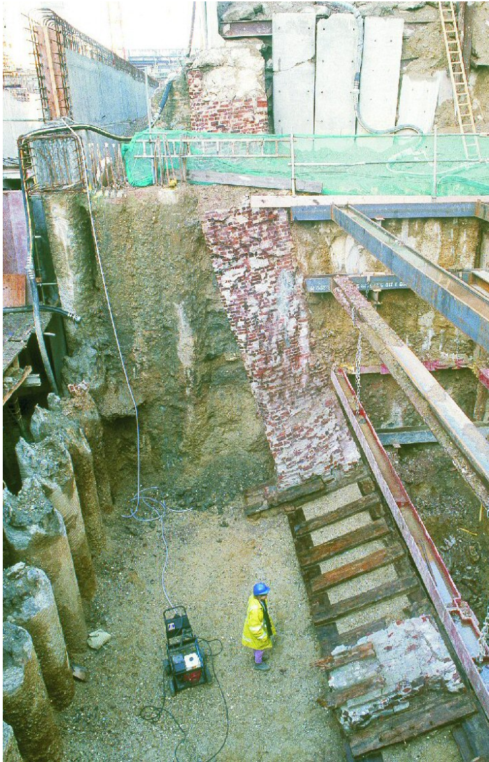
Figure 3 Curving brick wall supported by timber grillage (photograph MoLAS)
