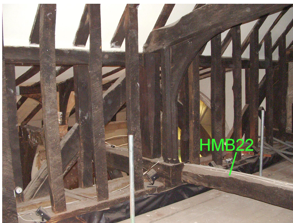
Figure 9: Inner nave, looking north-east, showing the tiebeam sampled
