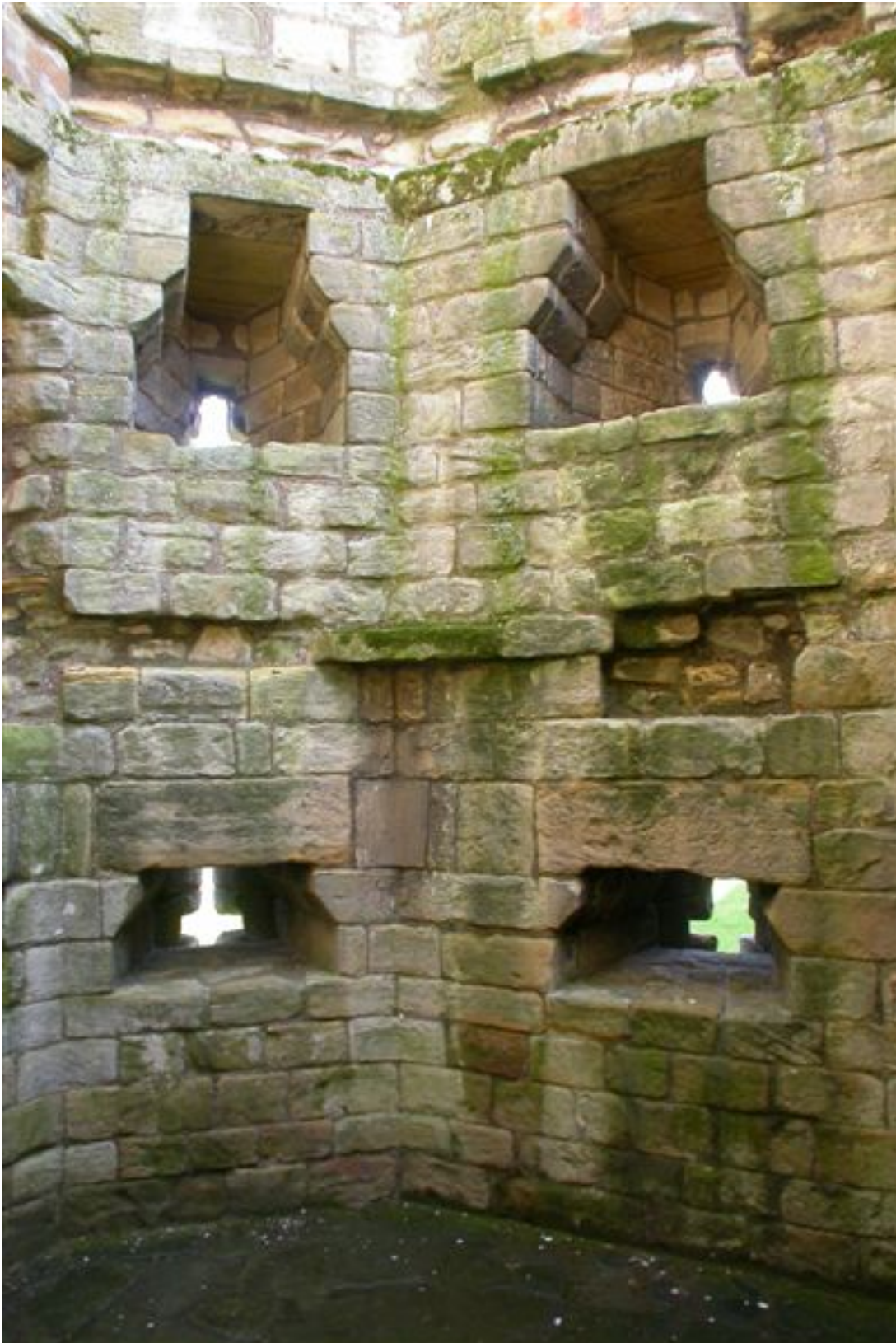
Figure 5: View of the slit windows with one of the accessible lintels (John Goodall)
