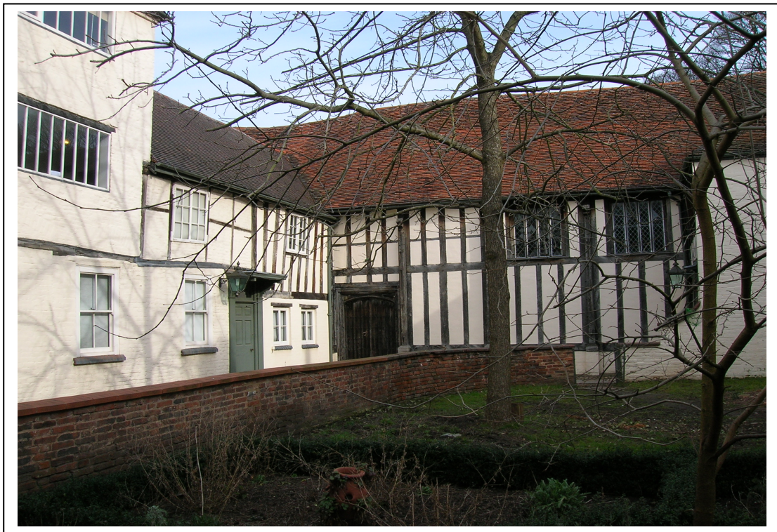
Figure 4a/b: East side of the infirmary wing and addition (above) and the south face of the Great Hall (below)
