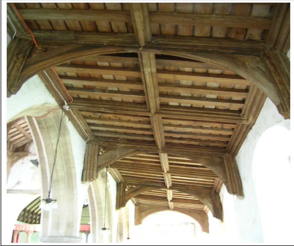
Figure 5: View of the south aisle roof looking west to east
