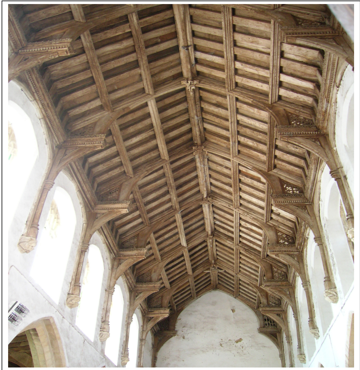
Figure 3: View of the nave roof viewed from the east looking west
