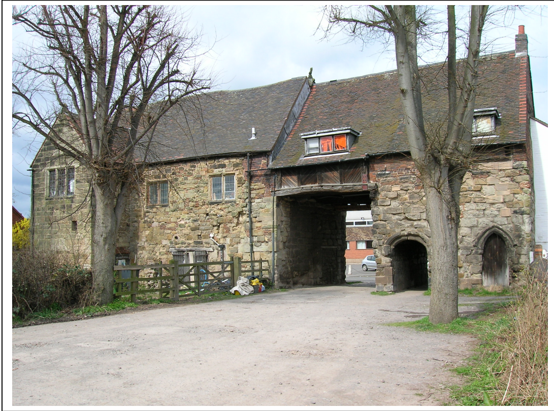
Figure 3: Rear, or south view of Polesworth Abbey Gatehouse, showing the Gatehouse proper (to the right) with its carriageway, pedestrian portal, and door of stairway to mezzanine and upper floor, and the annex to the left with its short gabled arm, possibly a porch or staircase
