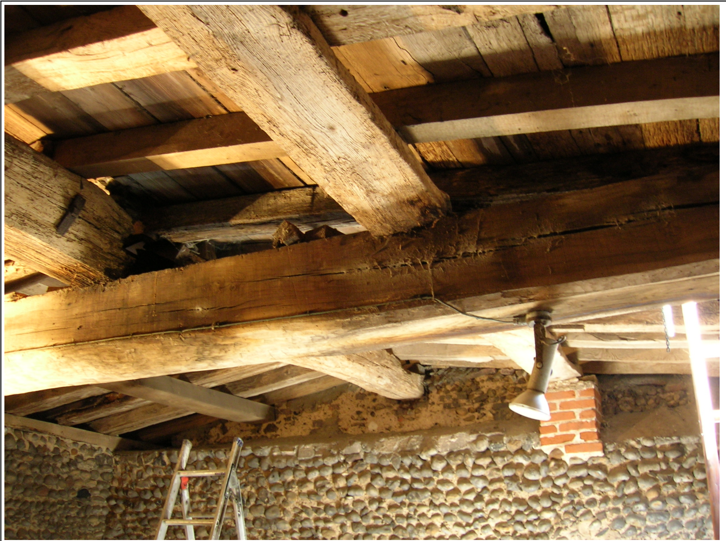
Figure 4: West tower roof, looking north-east
