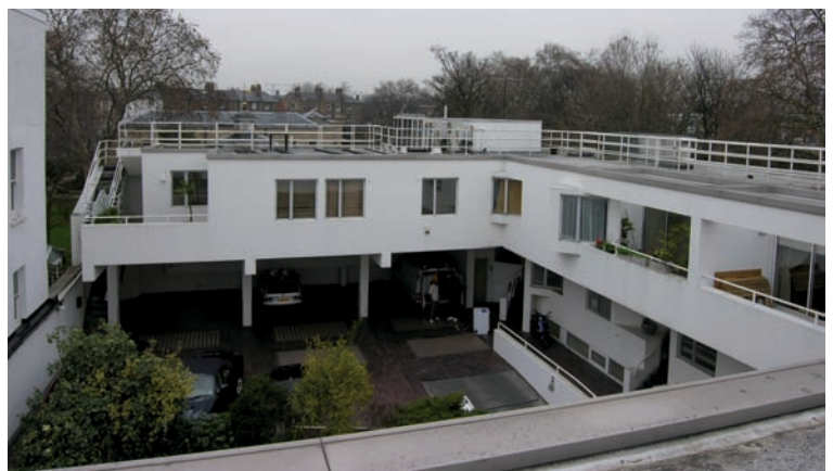
Fig. 3: View looking north from the roof (DP040009)
