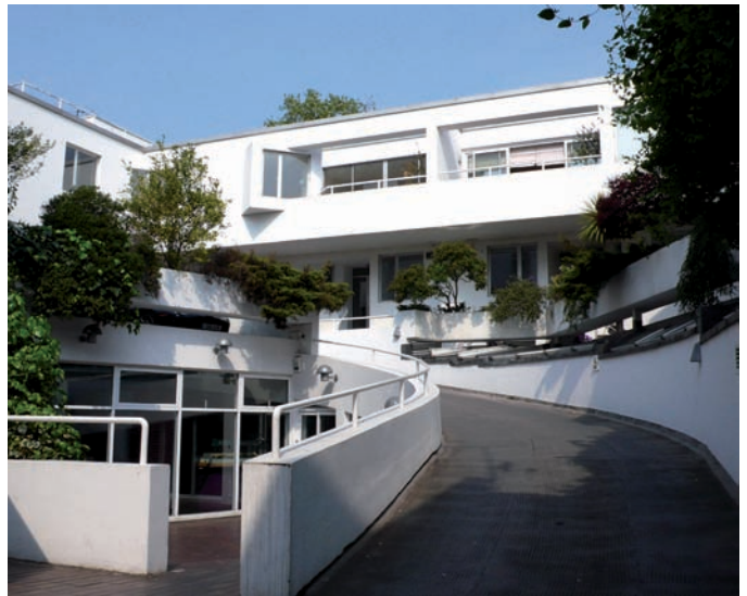
Fig. 1: View looking east, showing renewed (left) and inserted (right, under ramp) office fenestration (DP040021)
