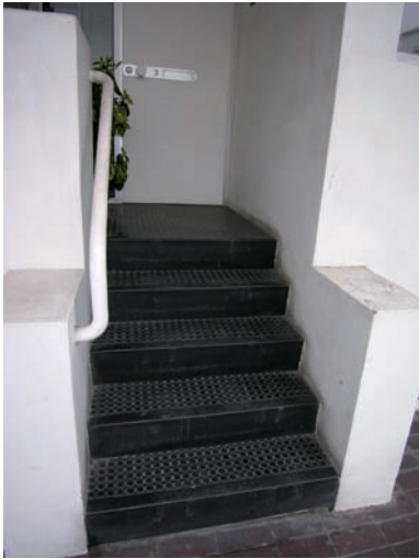
Fig. 20: Pirelli rubber matting in the apartment steps and porch (DP040014)
