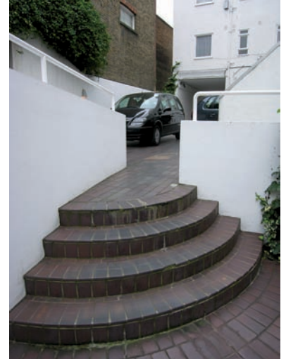
Fig. 22: Brick steps to offices (DP040016)
