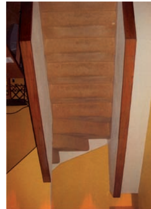
Fig. 14: Stairs to second floor (Jon Wright, © 20th Century Society)
