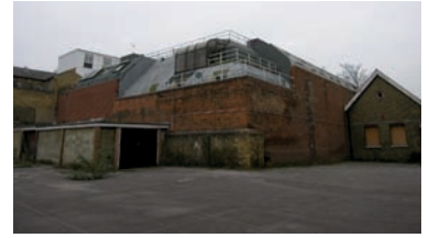
Fig. 4: The outer elevations viewed from the school playground (DP040020)
