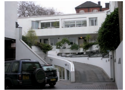
Fig. 7: The car ramp from the west (DP040019)
