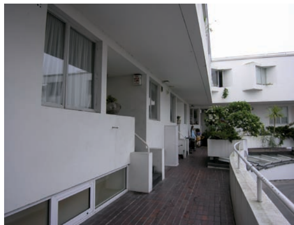
Figs 11 and 12: Views of the 'pedestrian deck' (DP040012; DP040015)
