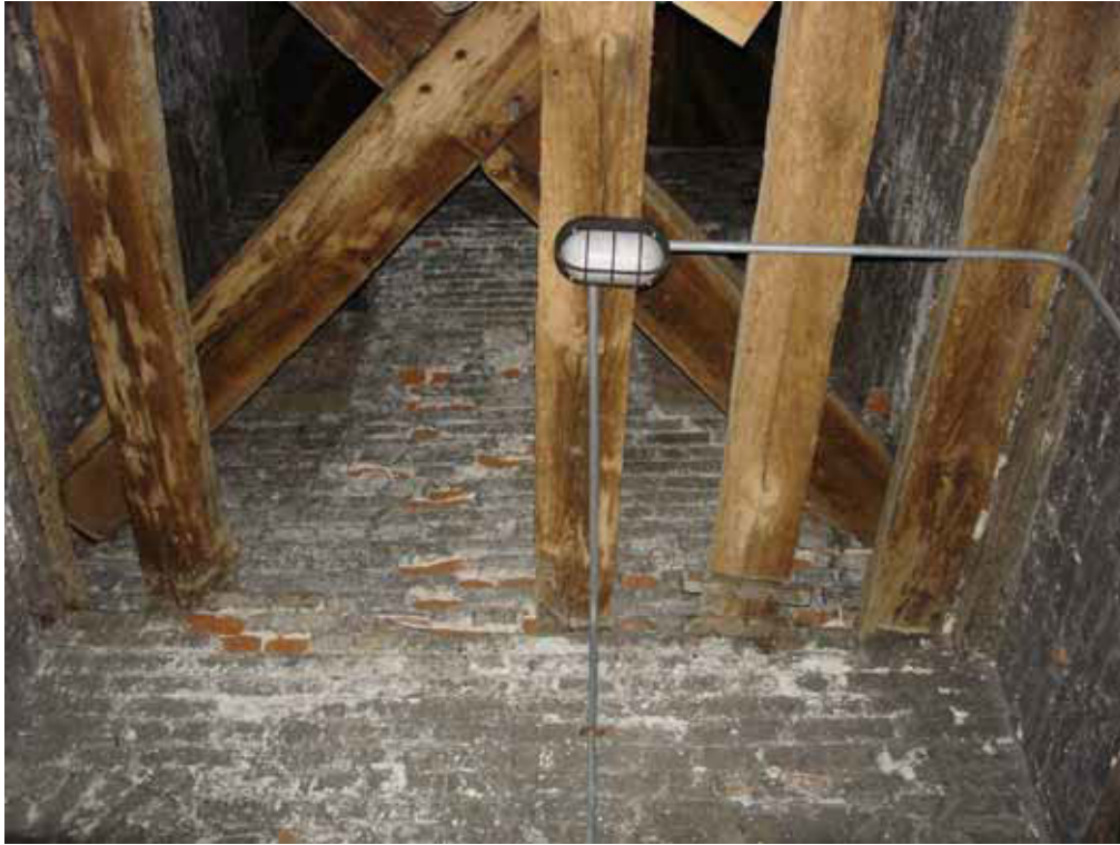
Figure 44: Second-floor details and cross-braces in south-west turret
