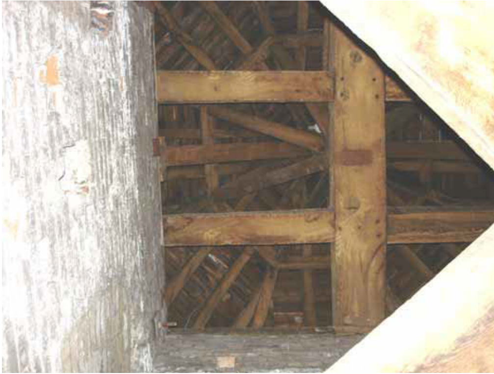
Figure 45: View of roof inside south-west turret
