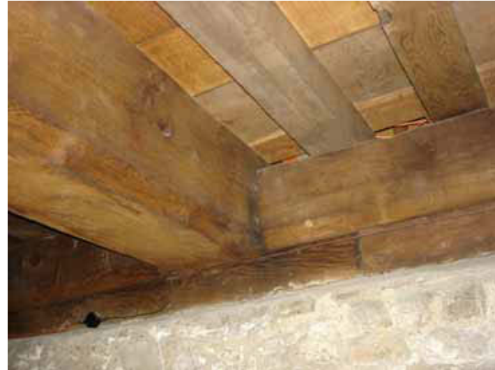
Junction of tiebeam and wallplates
