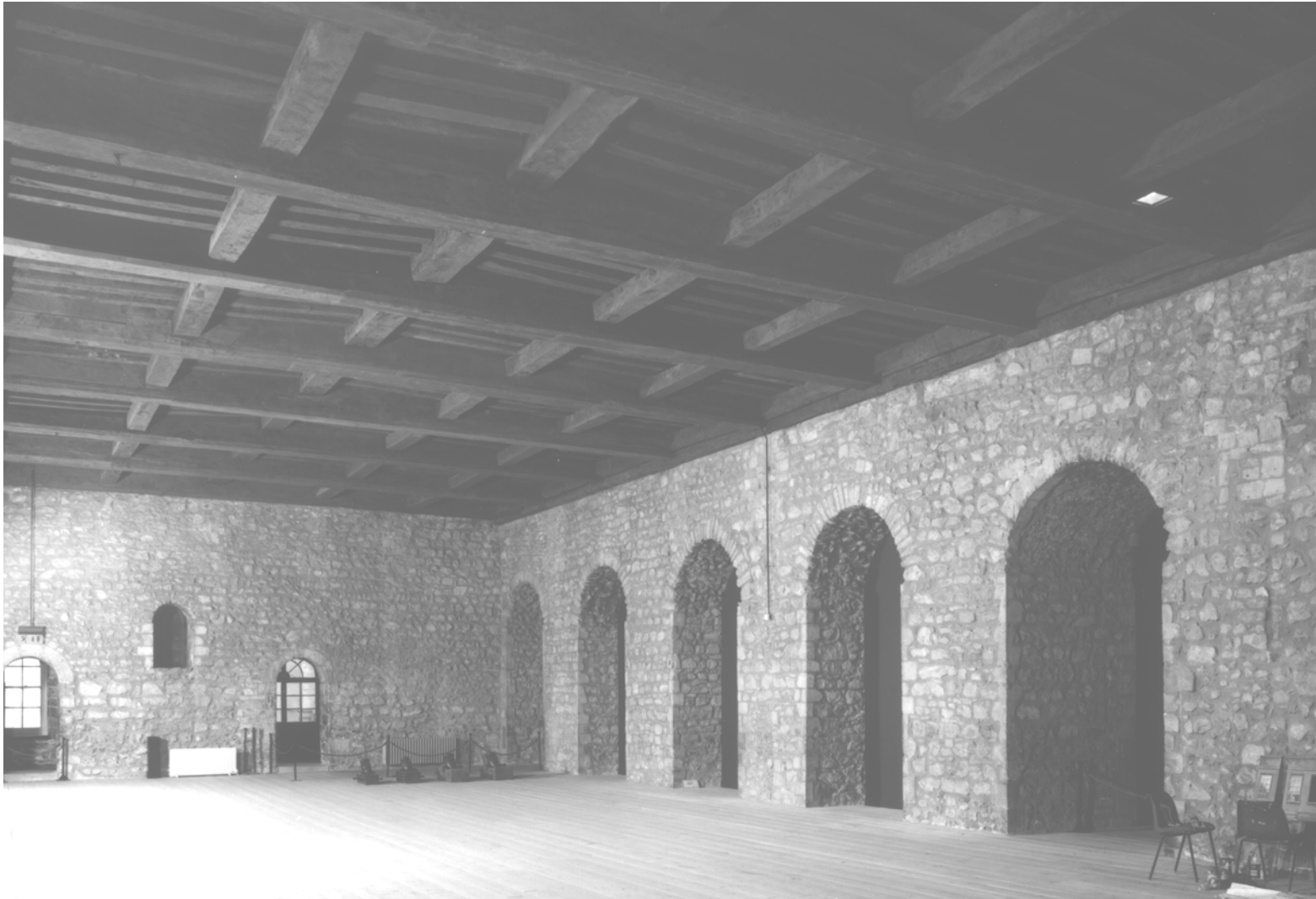
Figure 25: Photograph of western room roof (copyright Historic Royal Palaces)
