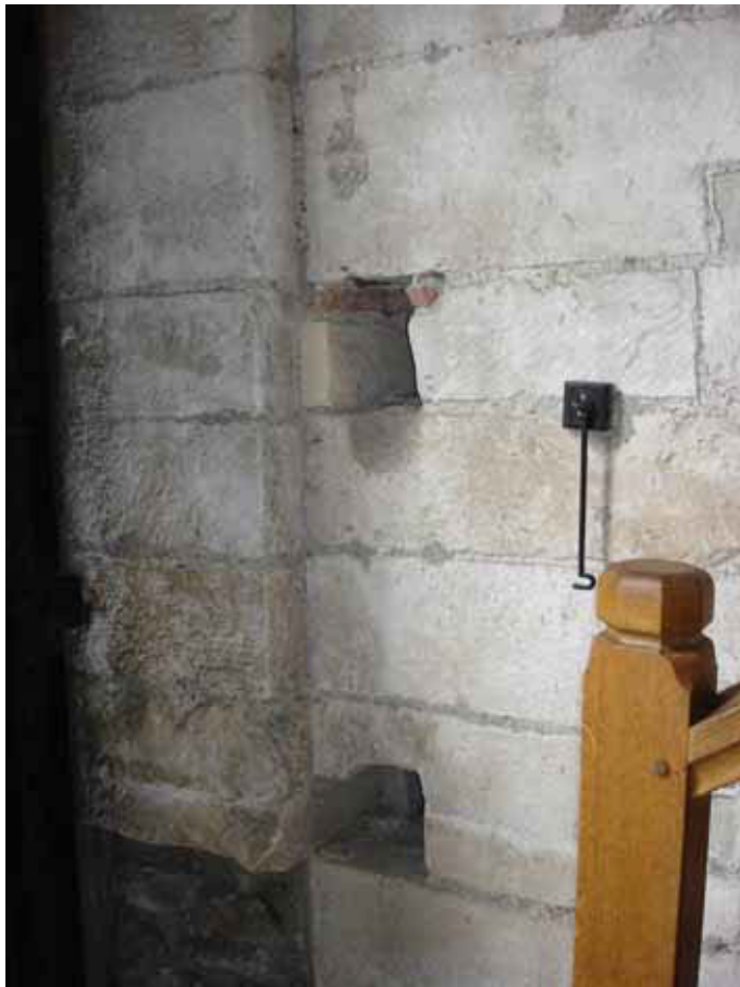
Figure 9: Door jamb and drawbar socket on west side of ground-floor entrance
