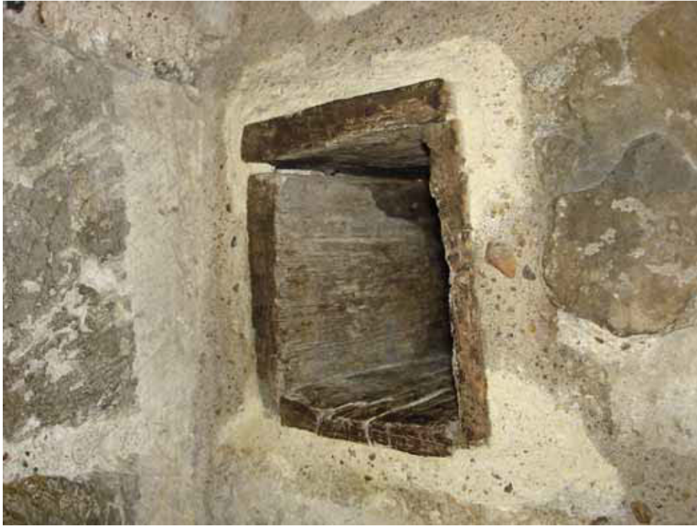
Figure 8: Drawbar socket in ground-floor spine wall (wt15–wt18)
