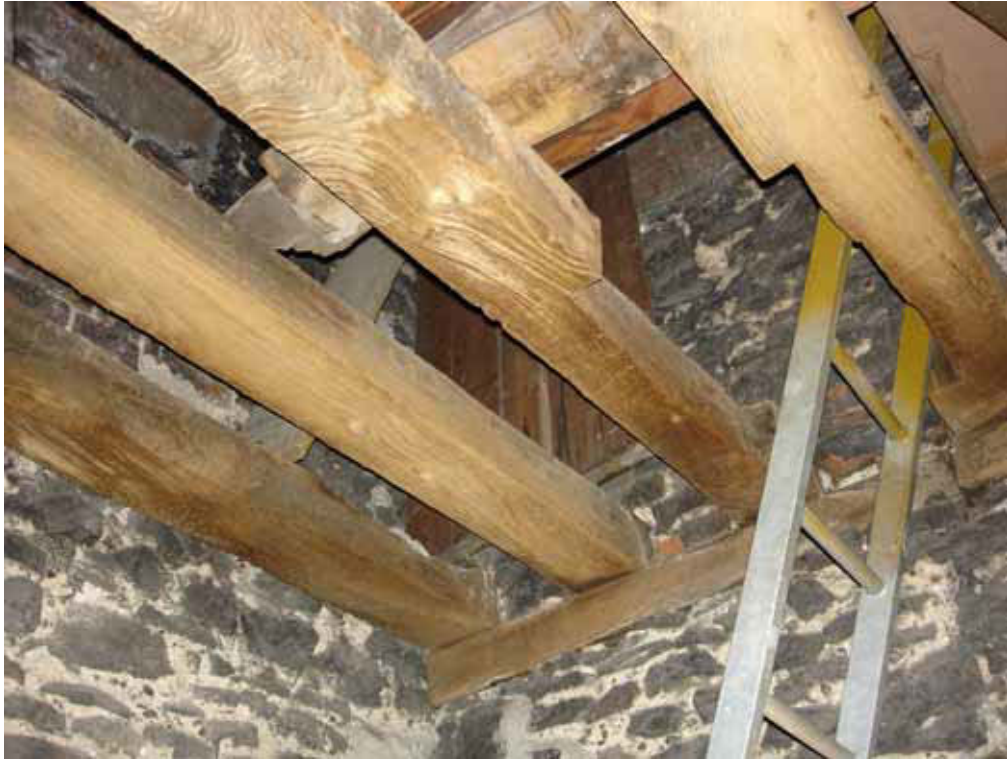
Figure 41: Second-floor details of south-east turret
