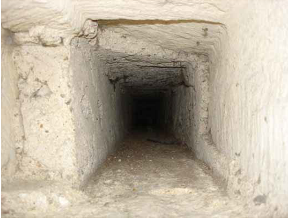
Figure 10: Detail of drawbar socket on west side of ground-floor entrance (wt08–wt14)
