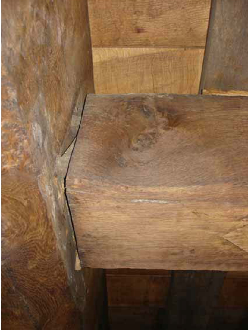
Junction of purlins and tiebeam
