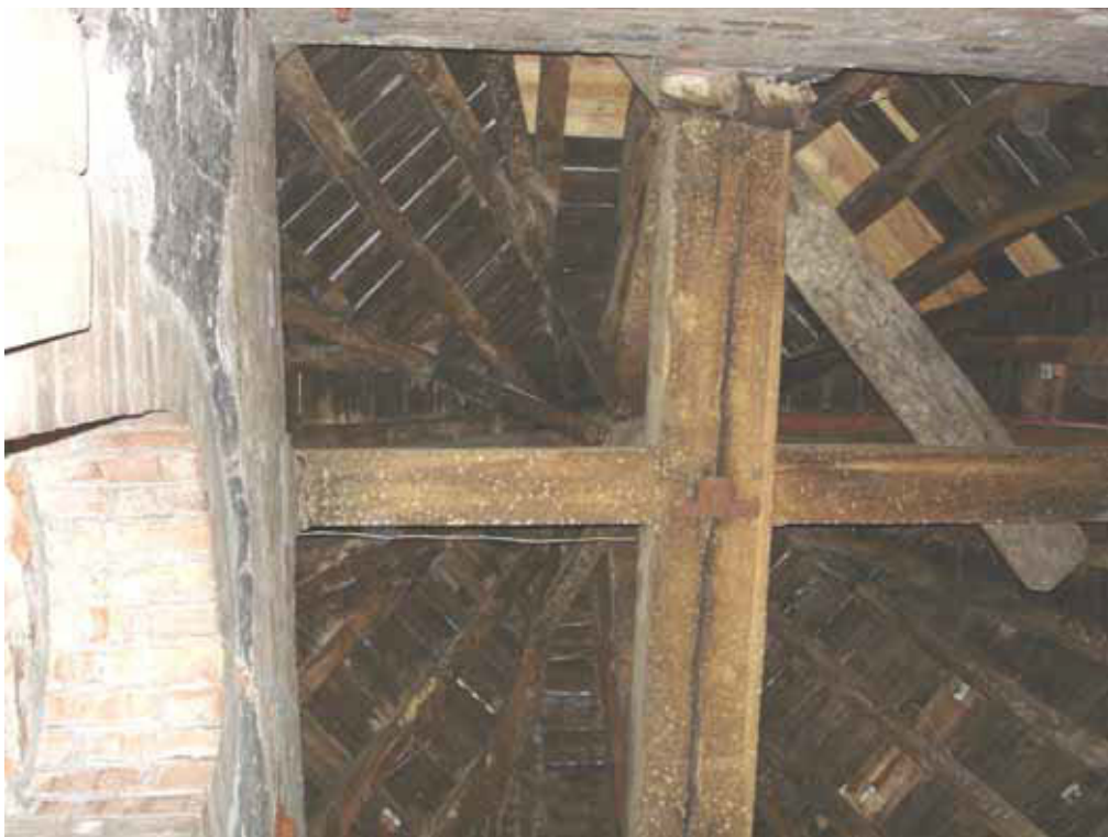
Figure 42: Underside of roof of south-east turret
