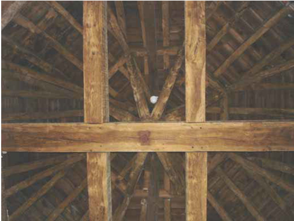
Figure 38: Roof, north-west turret
