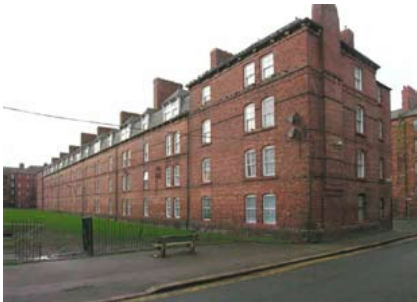
Fig 2: Tenement block to the rear of Devonshire buildings between Steamer Street and Sloop Street. (DPI46628)
