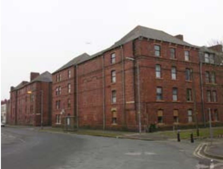
Fig 4: Egerton Buildings from the north. (DPI46629)
