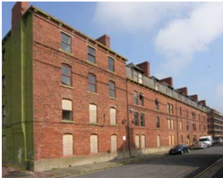
Fig 5: The Siemens Street elevation of the south-east block. (DPI46630)
