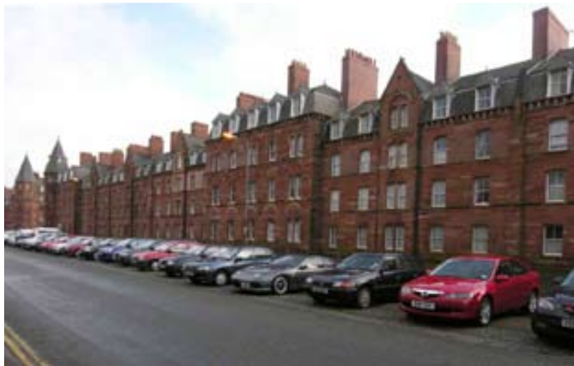
Fig 1: Devonshire Buildings, built in 1872-5, from Michaelson Road. (DPI46627)
