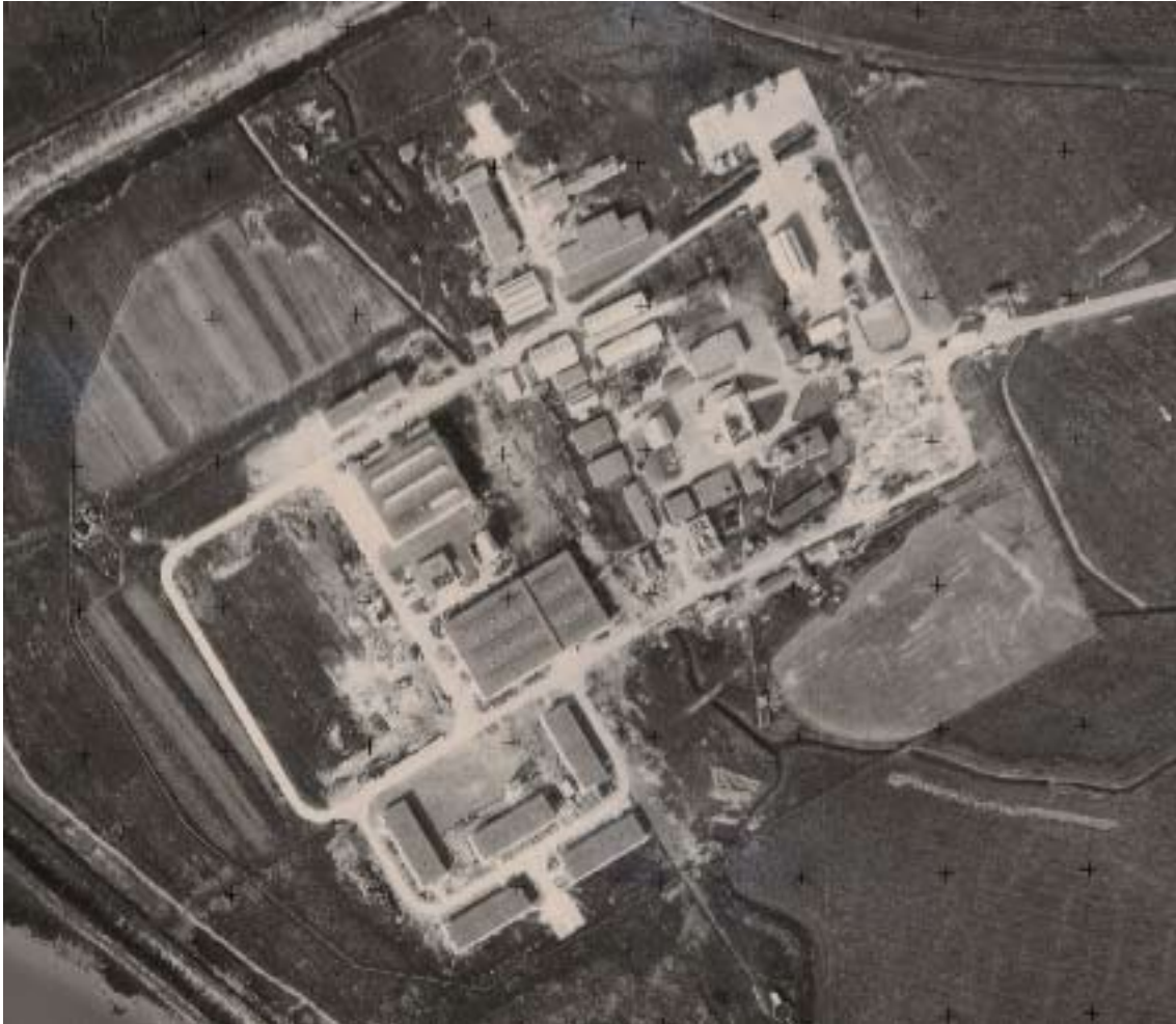
Figure 48: The Headquarters Area in July 1956 showing the post 1954 expansion to the west, east and north. (c) Crown copyright 58/2011 v 27 Jul 1956 0084
