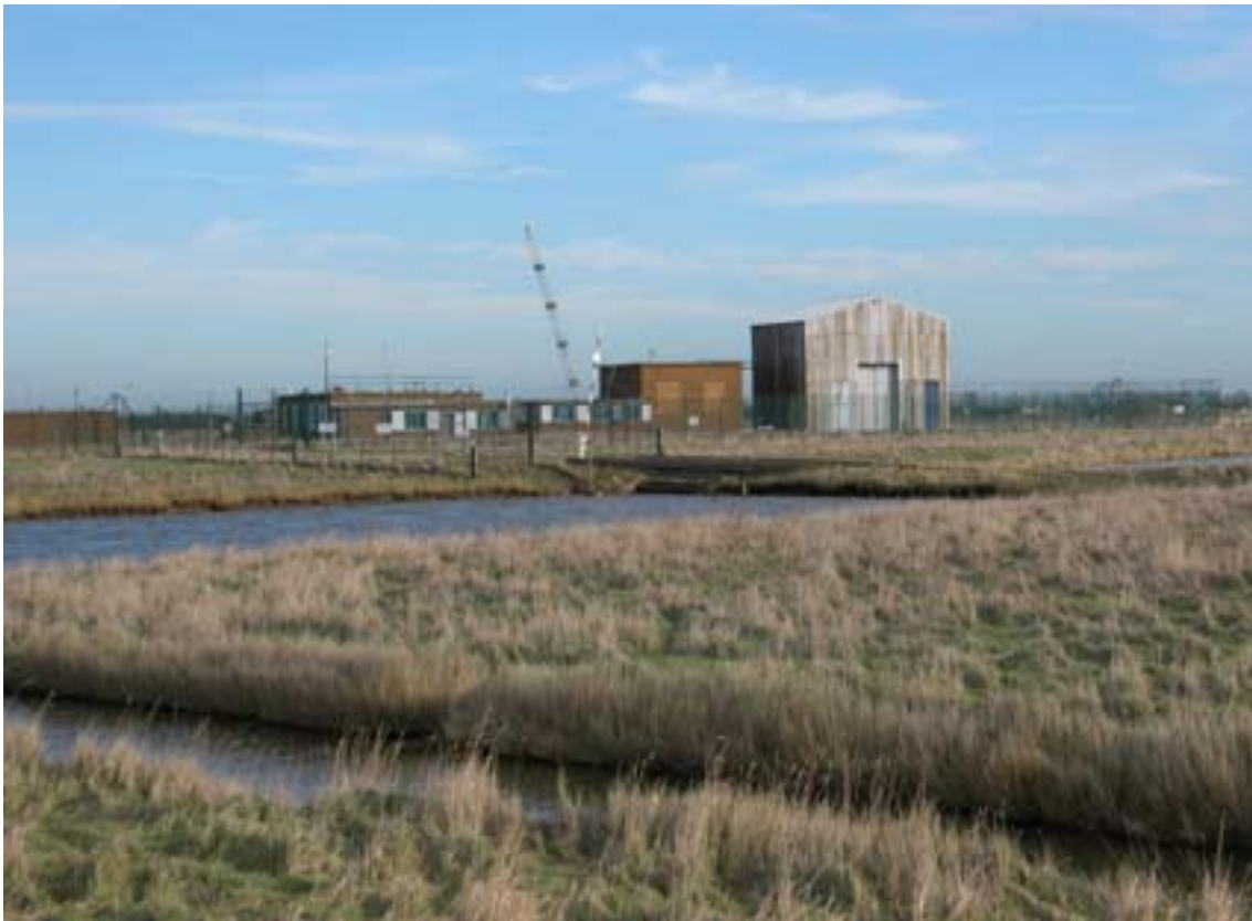
Figure 28: The Structures Laboratory from the southwest, in the centre is S5 the Concrete Laboratory and to its right S/SF11 the Pressure Test building . (c) English Heritage
