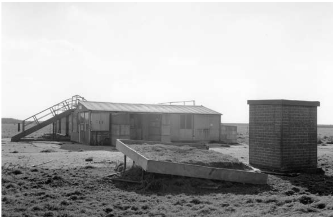
Figure 22: Large Area Open Range Thermal Simulator (LATS) or Thermal Radiation Facility J/SF20. To the rear is the building that housed the powdered aluminium and liquid oxygen bottles and to its rear the platform on which test equipment was mounted. In the foreground is the movable platform on which manikins were placed. (c) English Heritage BB99/15986
