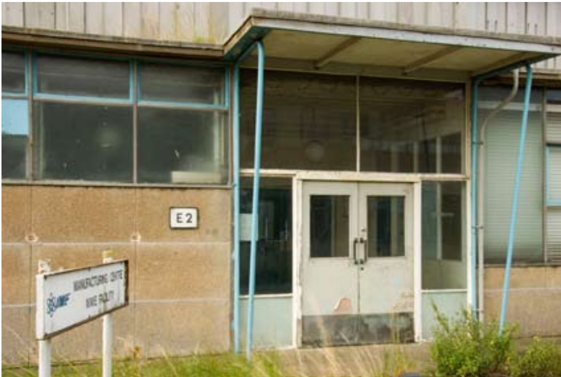
Figure 49: Main Mechanical Workshop E2, this building exhibits many features typical of the mid-1950s structures, including the hung concrete wall panels, Crittall windows, pressed aluminium sheet cladding and a porch canopy supported by a tubular steel framework. (c) English Heritage DP035959
