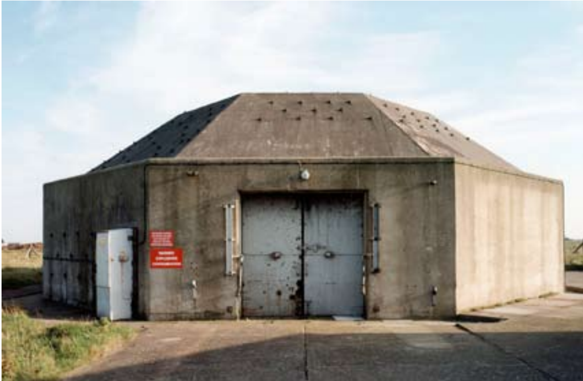
Figure 32: 1970s Fragmentation Control Building N14. (c) English Heritage BB99/15975
