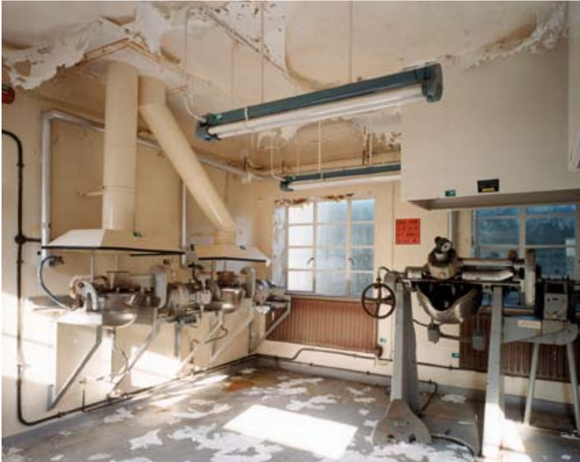
Figure 41: Casting Shop X10, was 56, showing the steam heated jacketed mixing bowls used to melt and cast high explosives. (c) English Heritage BB99/15981
