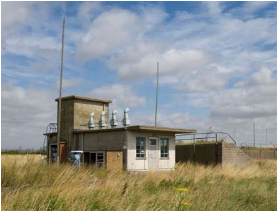
Figure 40: Casting Shop X10, was 56, built about 1953, with a rear reinforced concrete wall and to the right is later breeze block and earthwork traverse. (c) English Heritage DP035931
