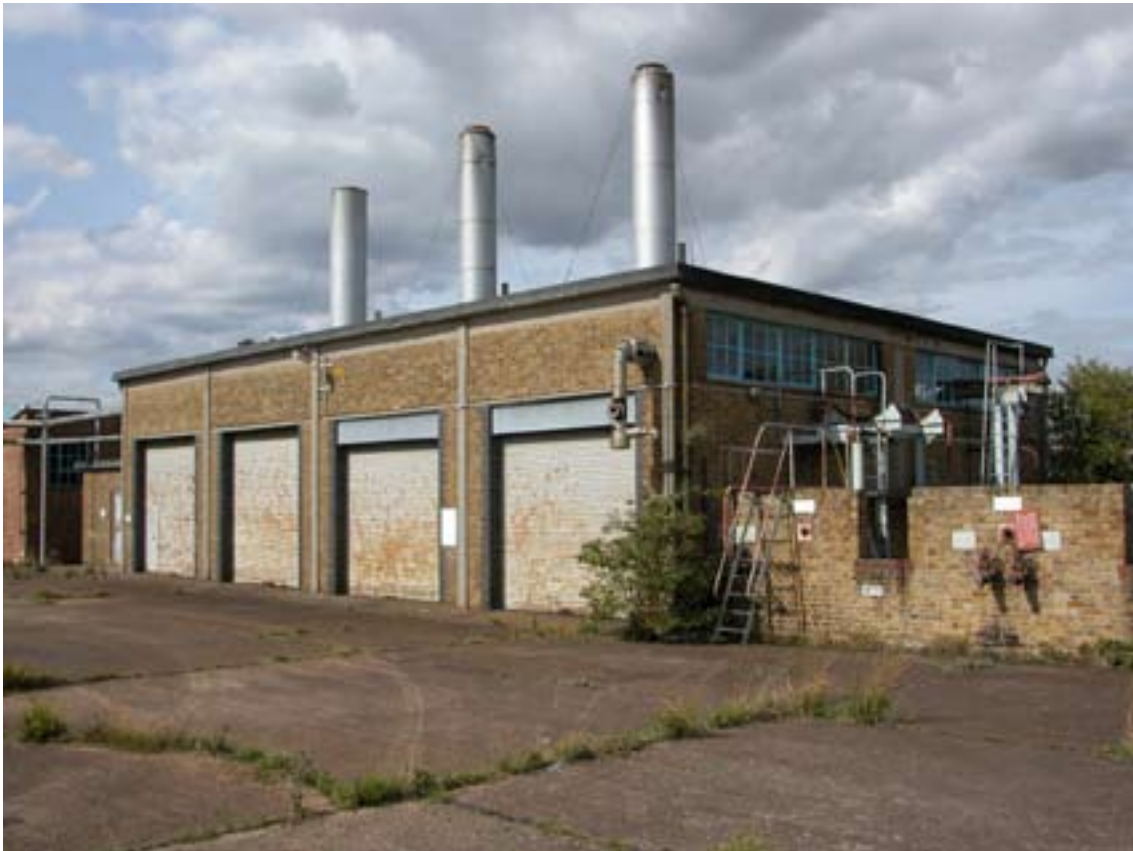
Figure 55: Boiler House E4. (c) English Heritage
