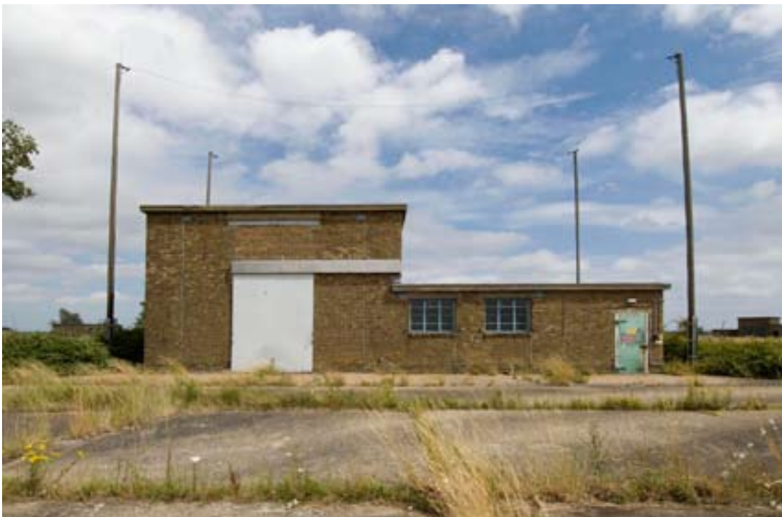
Figure 5: Explosives Preparation Laboratory X6, was 23, late in 1947 Superintendent Roy Pilgrim respecified the design of this building for its role in the atomic bomb project. In 1952, the United Kingdom's first live atomic device was assembled in this building. (c) English Heritage DP035925
