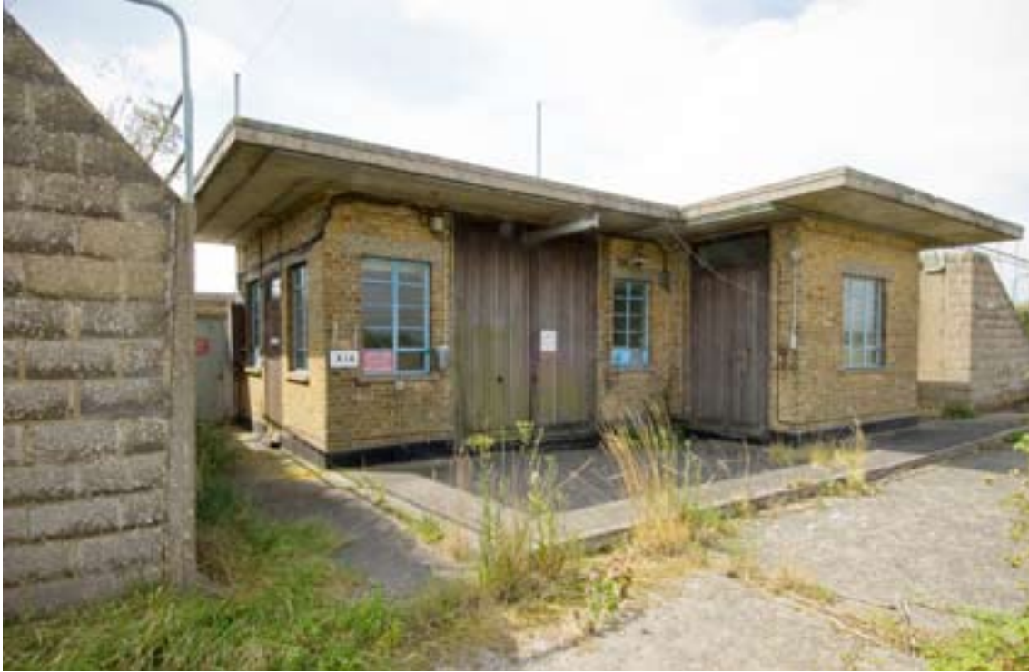
Figure 42: Explosives Machining shop X13 built about 1955, this group of buildings were distinguished by well-finished brickwork, gravel washed lintels and sills, and teak doors. To either side are later breeze block and earthwork traverses. (c) English Heritage DP035934
