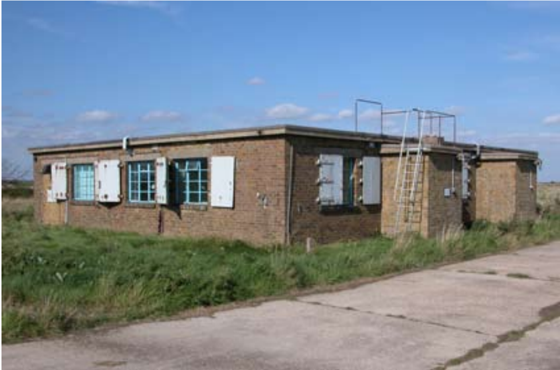
Figure 17: Office and Laboratory 13, this building is typical of the late 1940s and early 1950s range control buildings with brick walls, a flat concrete roof and steel Crittall windows protected by hinged steel shutters. (c) English Heritage
