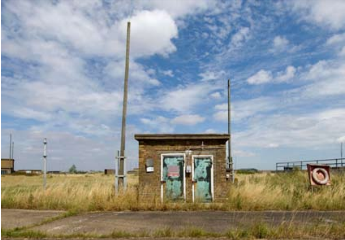
Figure 35: Special Store 22, now Magazine X3, was built in 1947, typical of this date is its brick construction and copper clad doors. Characteristic of explosives buildings are the lightning conductors, copper earth straps and external electrical fittings. DP035923 (C) English Heritage
