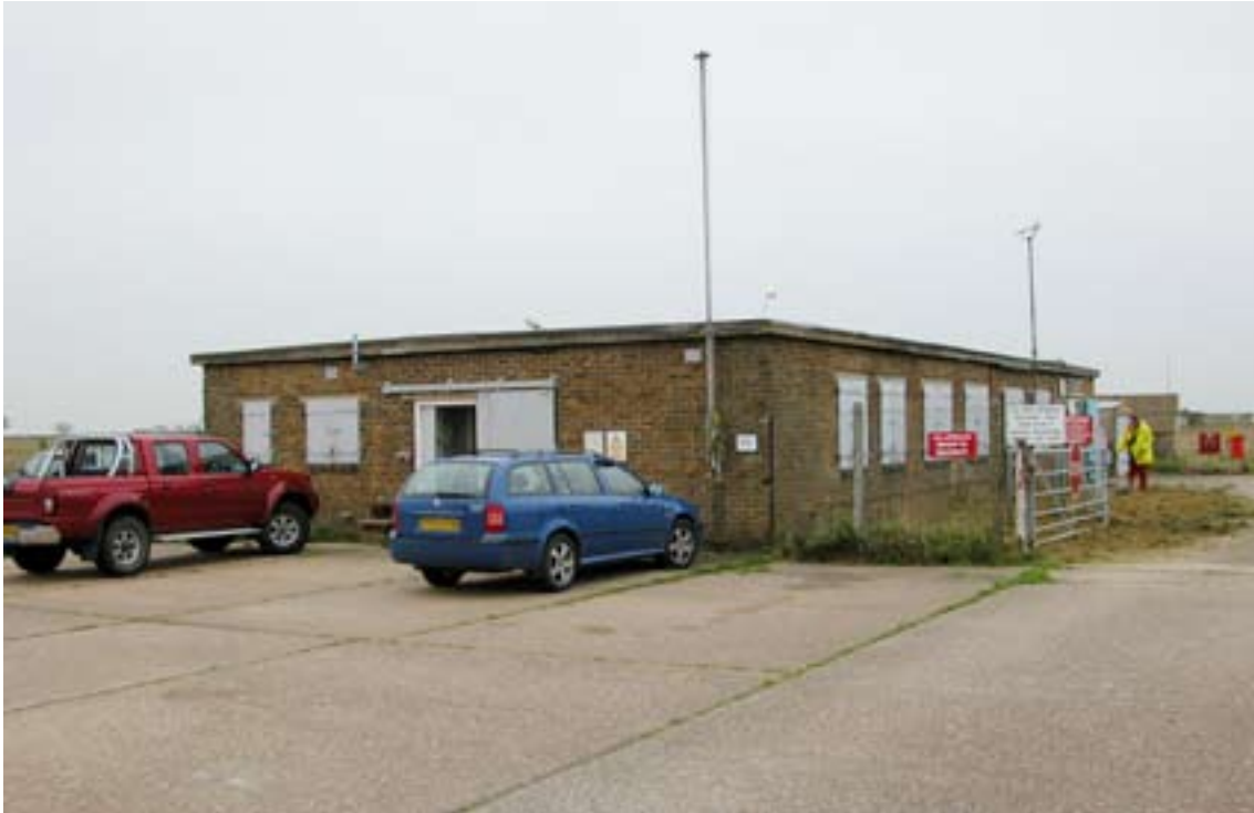
Figure 12: Office and Electronics Laboratory F1. (c) English Heritage
