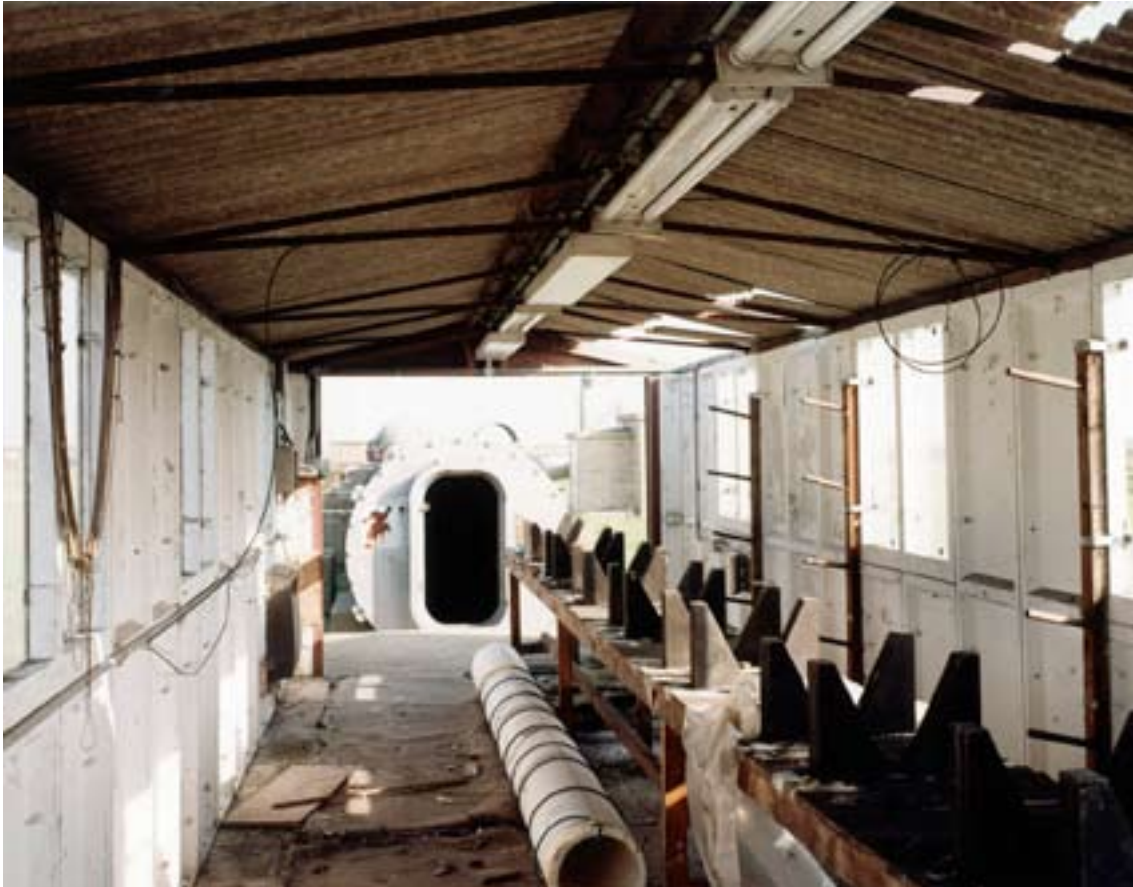
Figure 16: Charge Assembly Building I/SF46, this view shows the polystyrene former around which a length of detonating cord was wrapped. Once assembled the charge was suspended in the tunnel and the bulkhead doors sealed. (c) English Heritage BB99/16000
