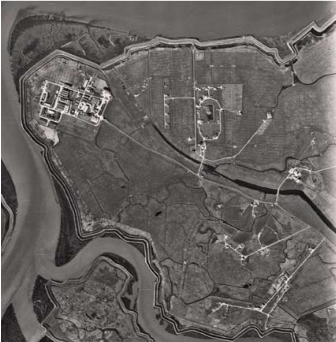
Figure 1: Air photograph showing most of AWRE Foulness in 1970, to the top is the River Roach and to the left Shelford creek and the Middleway. UNT HSLEssex 0387 16 Sept 1970
