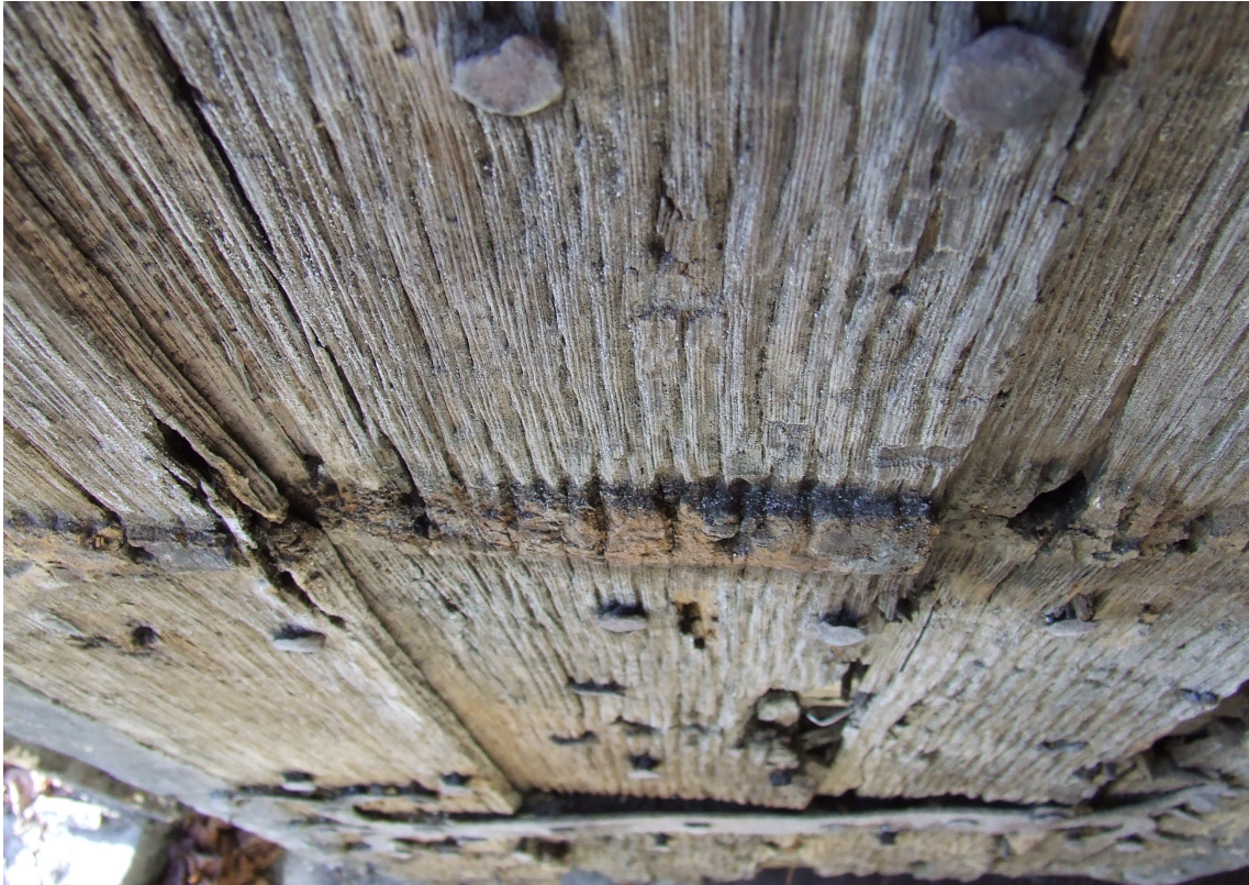
Figure 5. View looking down the outer face of the door from an elevated position, showing the degree of weathering and a raised section where ironwork once sat, protecting the wood surface
