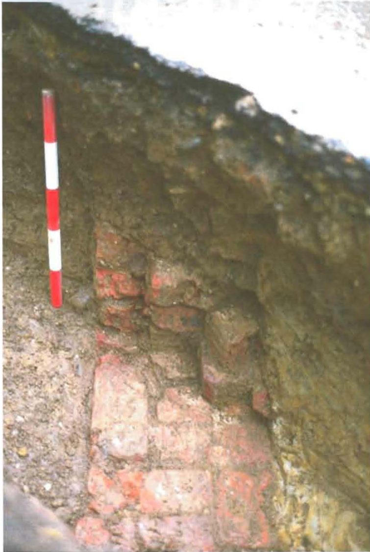
Figure 8. Trench 1, remains of 18th century stable block wall looking northwest
