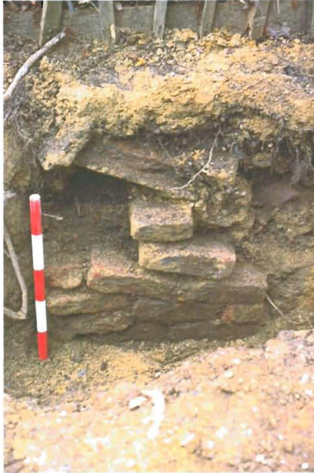
Figure 6. Photograph of context 101 - one of the three brick structures seen in the excavations along the side of the road in trench 1 to the north-west of the house
