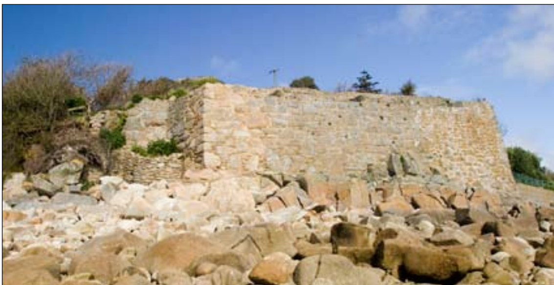
Figure 22. Lower Benham Battery showing the repairs it has undergone [DP022418]
