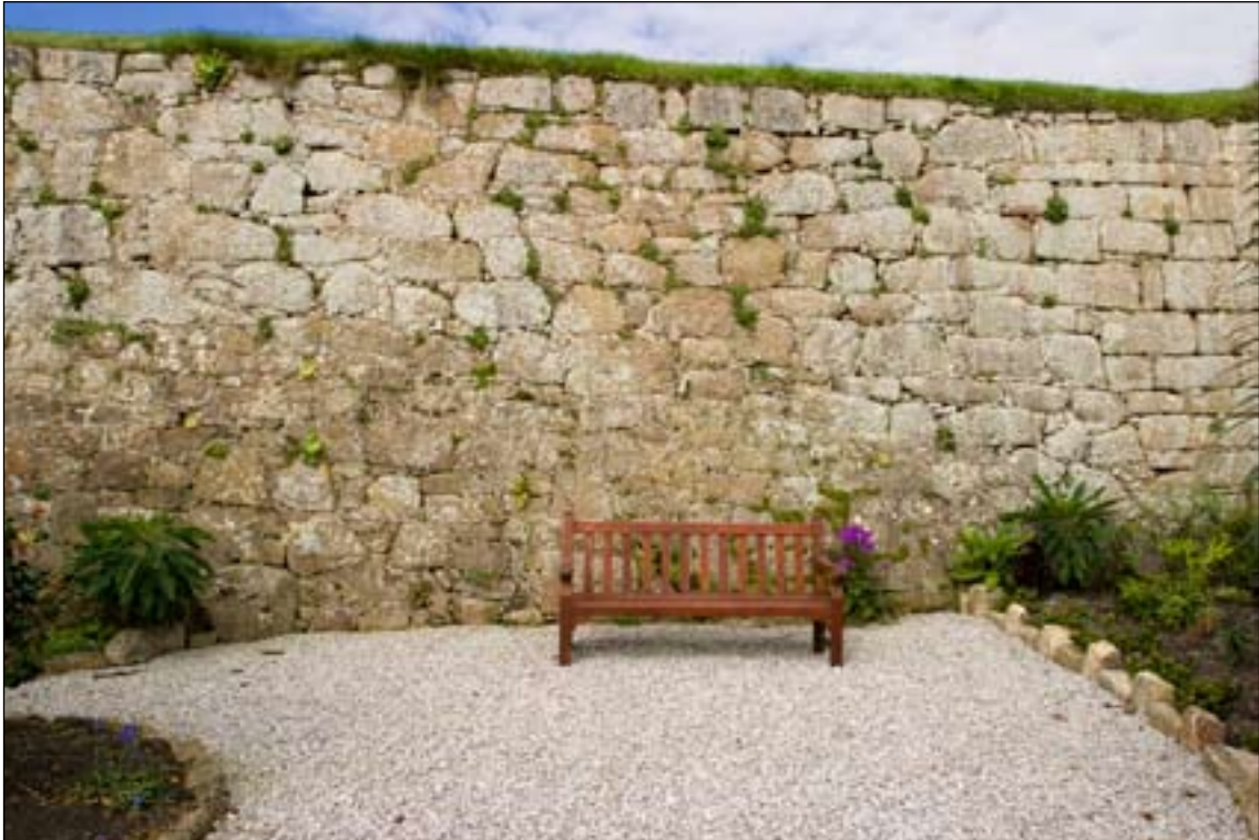
Figure 13. Wall to south of Garrison Gate [DP022358]
