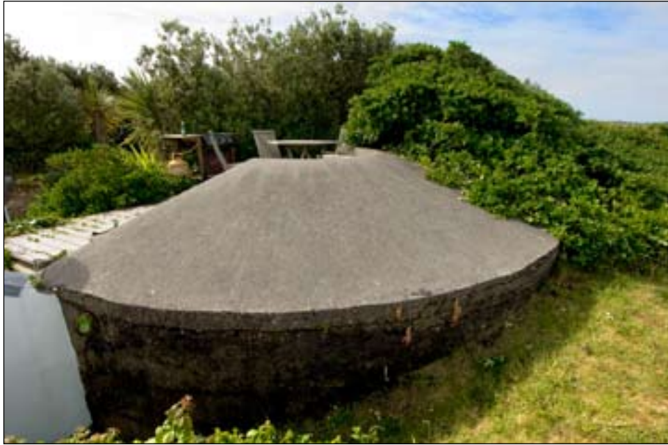
Figure 45. Steval Point Quick-Firing Gun Battery – position of gun [DP085183]
