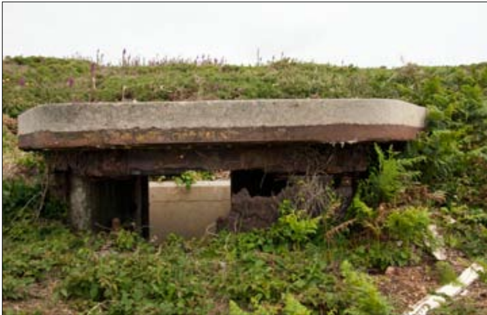
Figure 44. Position Finder Station [DP085220]
