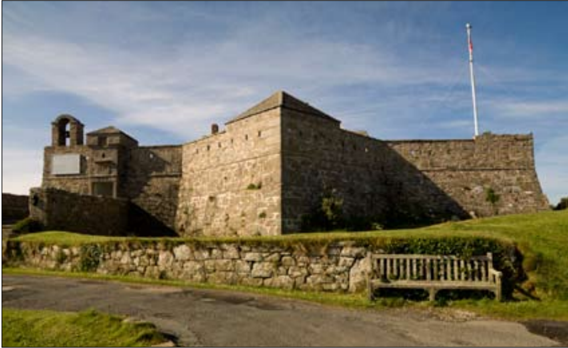
Figure 10. Star Castle North Elevation [DP085292]
