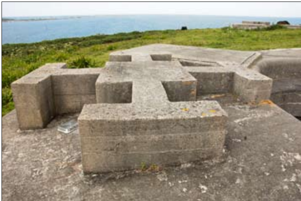
Figure 47. 'RACON' Beacon location on Woolpack Battery [DP085199]
