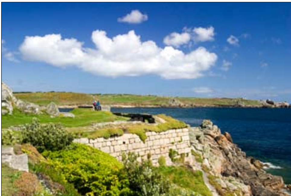
Figure 33. Morning Point Battery [DP022526]
