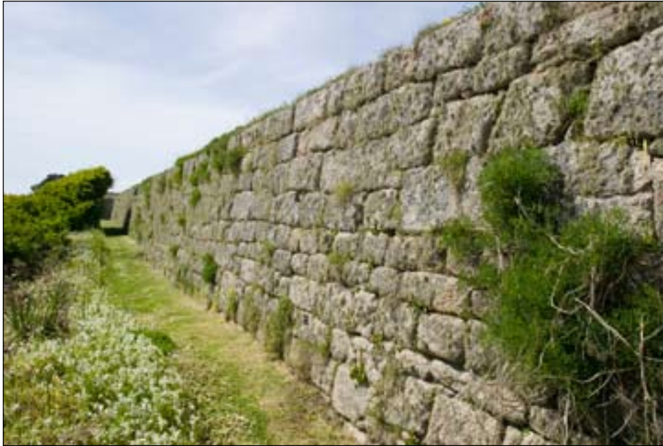
Figure 32. Wall to the west of Morning Point [DP022527]
