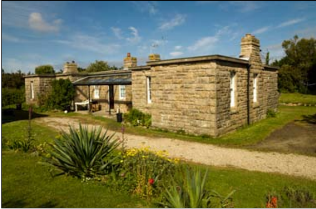
Figure 41. The Barrack Block between Woolpack and Steval Batteries. [DP085319]
