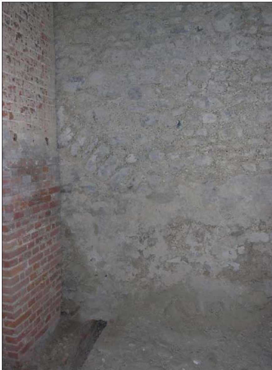
Figure 7. Line of voussoirs at upper end of hall
