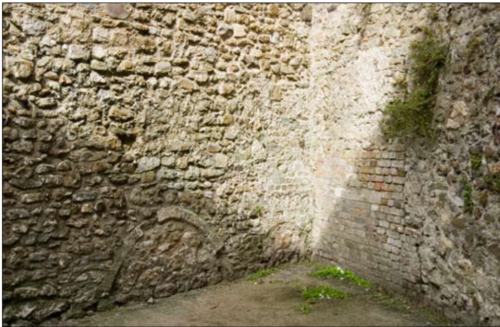
Figure 14. Blocked arches in corner of possible 'kitchen' at 13th-century floor level
