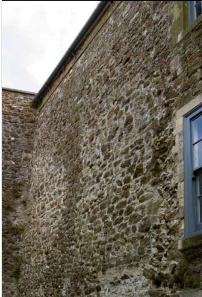
Figure 13. Outlines of roof line and former central division in upper storey
