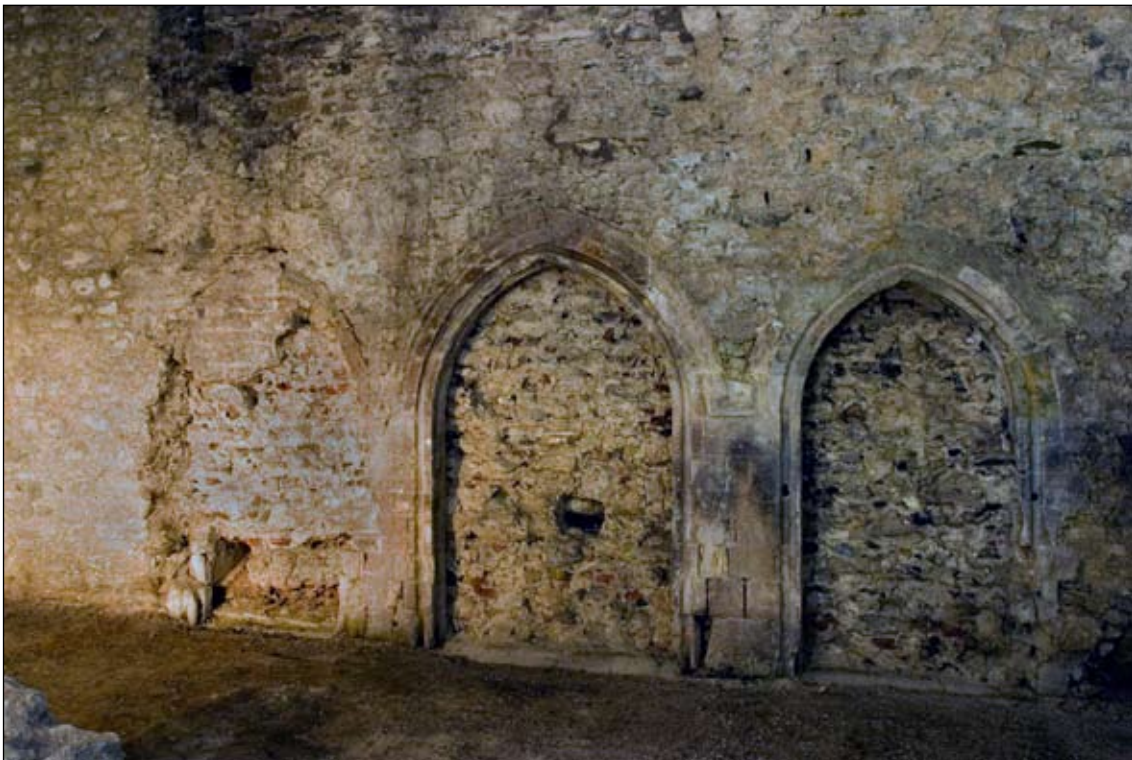
Figure 8. Service doorways at lower end of hall
