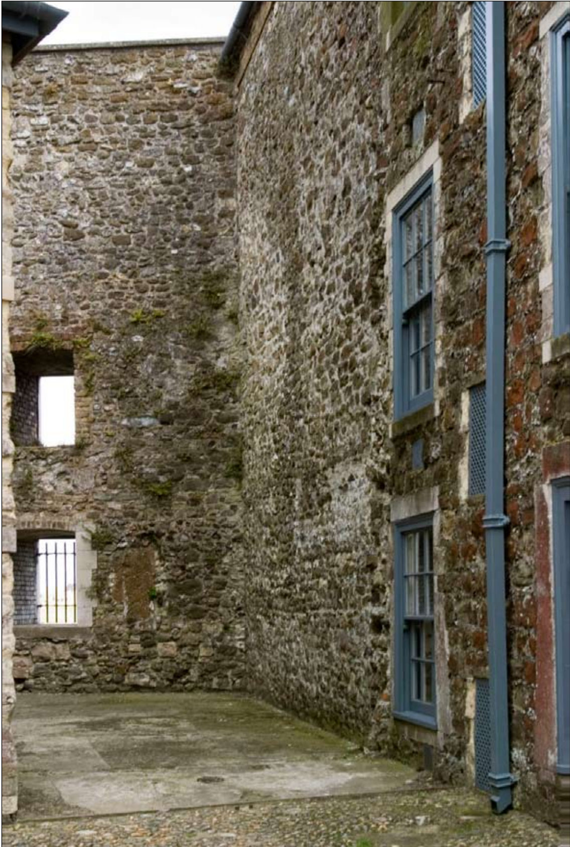
Figure 11. Site of former building interior (to left of sash windows)
