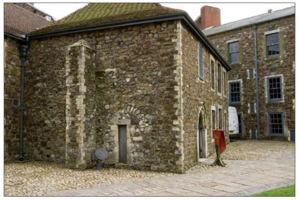
Figure 11. North-west wall of AV Building showing joint (at right side of end wall) between medieval rubble and regular 18th-century walling
