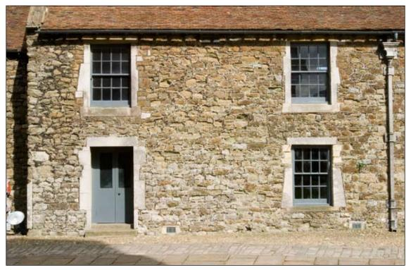
Figure 10. Joint between medieval rubble and regular 18th-century walling, to the left of the right-hand sashes
