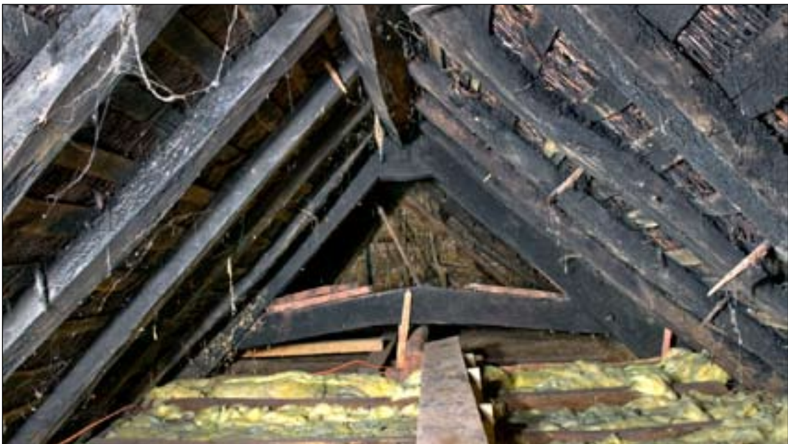
Figure 2. Roof space looking east towards cruck D-D1 showing smoke-blackened timbers and thatch (DPI13795).
