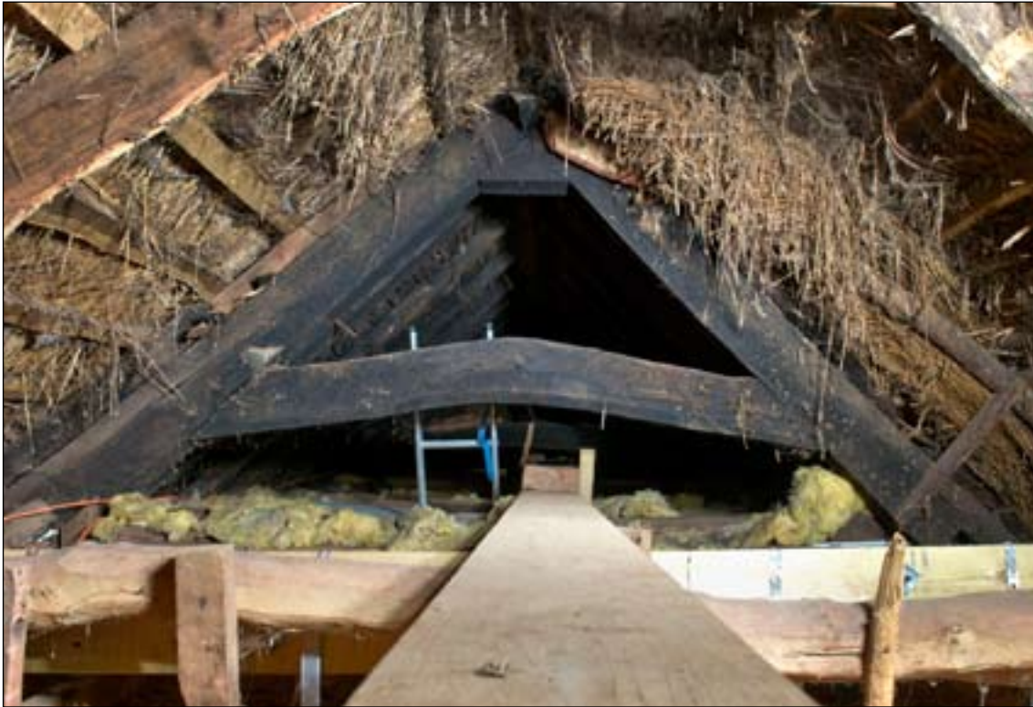
Figure 3. West face of cruck truss C-CI, also showing replaced timbers in Bay B-C (DPI13794).
