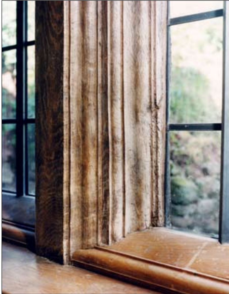
Figure 19. Detail of window-frame moulding of king mullion in window of north wing, ground floor (AA97101518).
