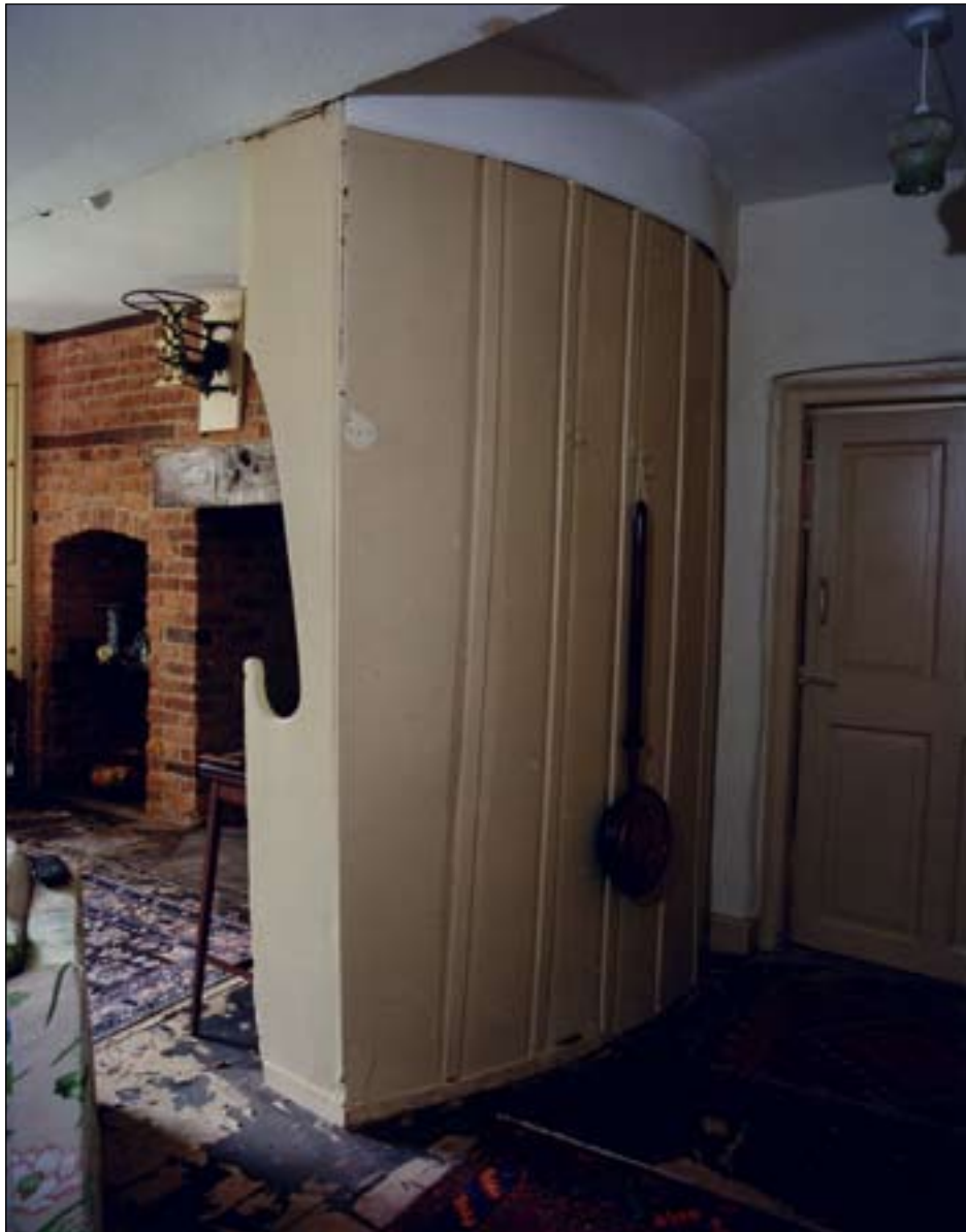
Figure 27. Interior of ground floor showing inserted brick chimney stack opening onto hall along B-B1, and settle (AA97/01519).
