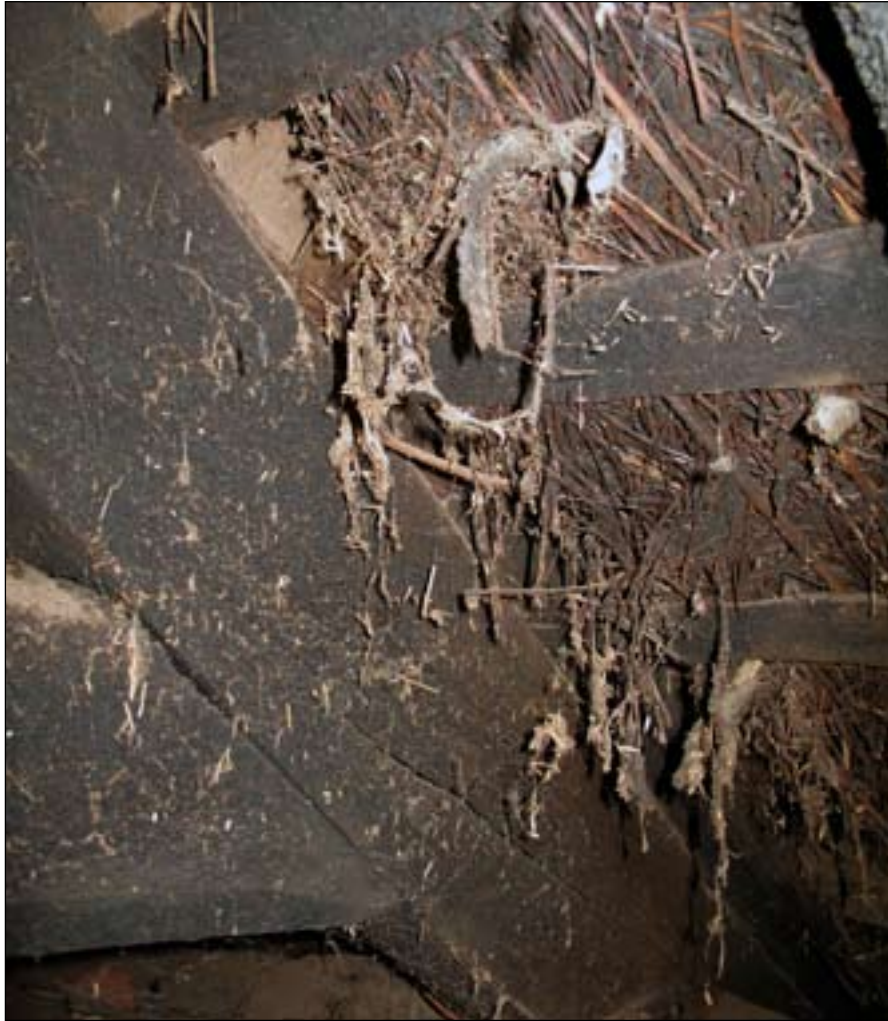
Figure 8. Detail of cruck C-CI, showing smoke encrustation and run-out stop on soffit of collar (DPI13781).
