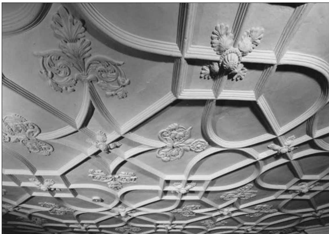
Figure 22. Plasterwork ceiling in ground-floor room of north wing (BB96/03908).
