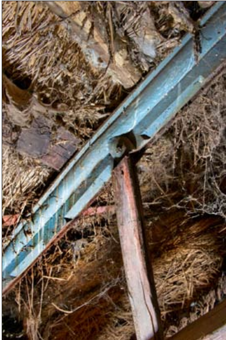
Figure 13. Section of medieval screen bressumer re-used as a rafter (DPI13793).
