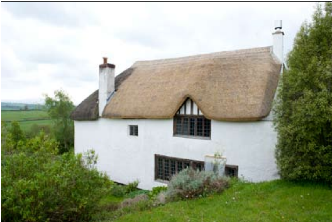
Figure 18. Exterior view from north-east showing small timber-framed gable (reconstructed in 1980s) above mullioned timber windows of north wing (DPI13772).
