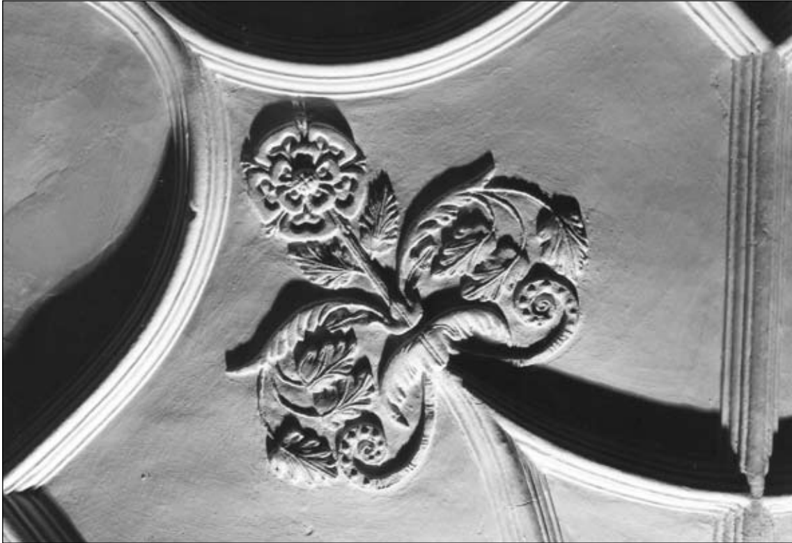
Figure 23. Detail of plasterwork ceiling in ground-floor room of north wing (BB96/03909).
