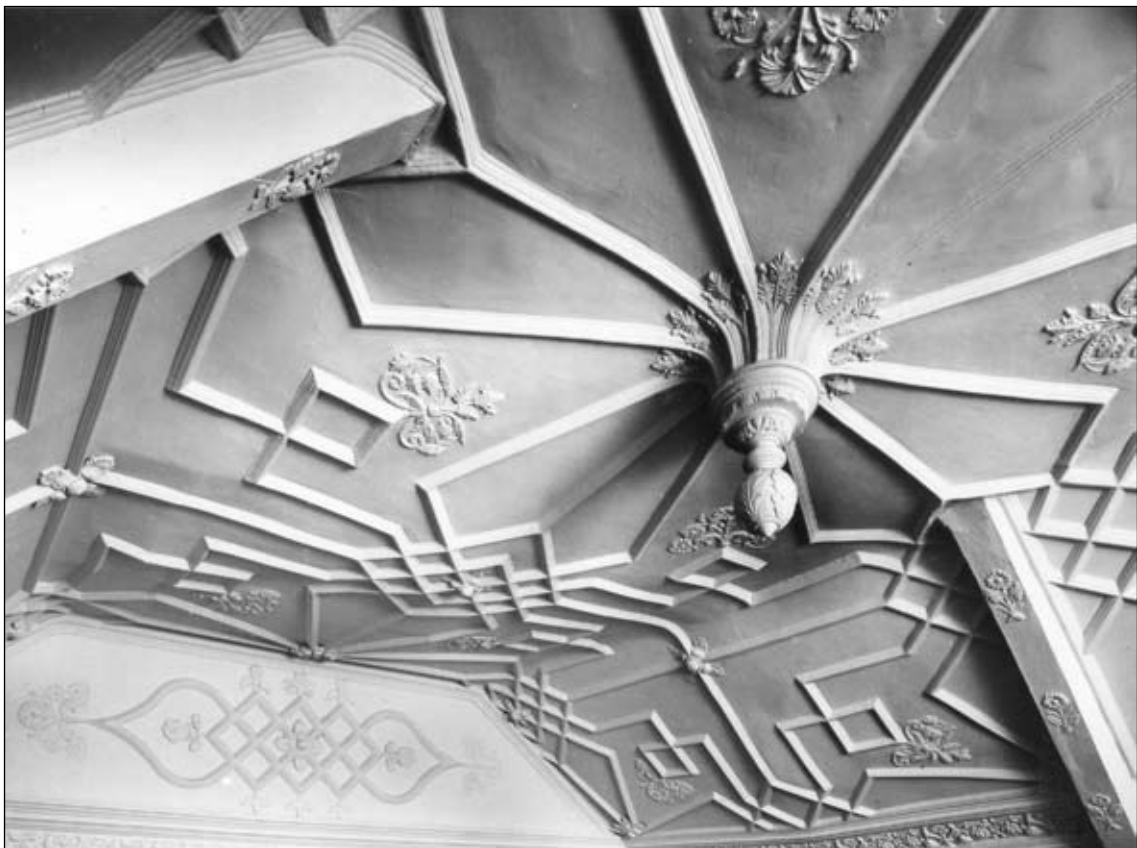
Figure 24. Plasterwork ceiling in first-floor room of north wing (BB96/03913).
