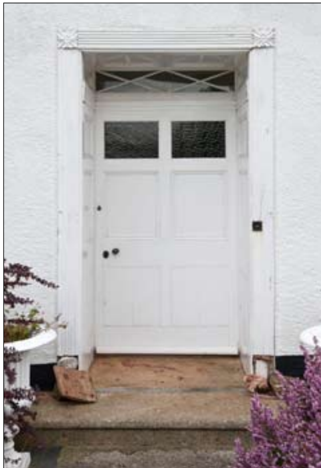
Figure 29. Regency-style doorcase inserted into facade at east end of main range (DPI13775).
