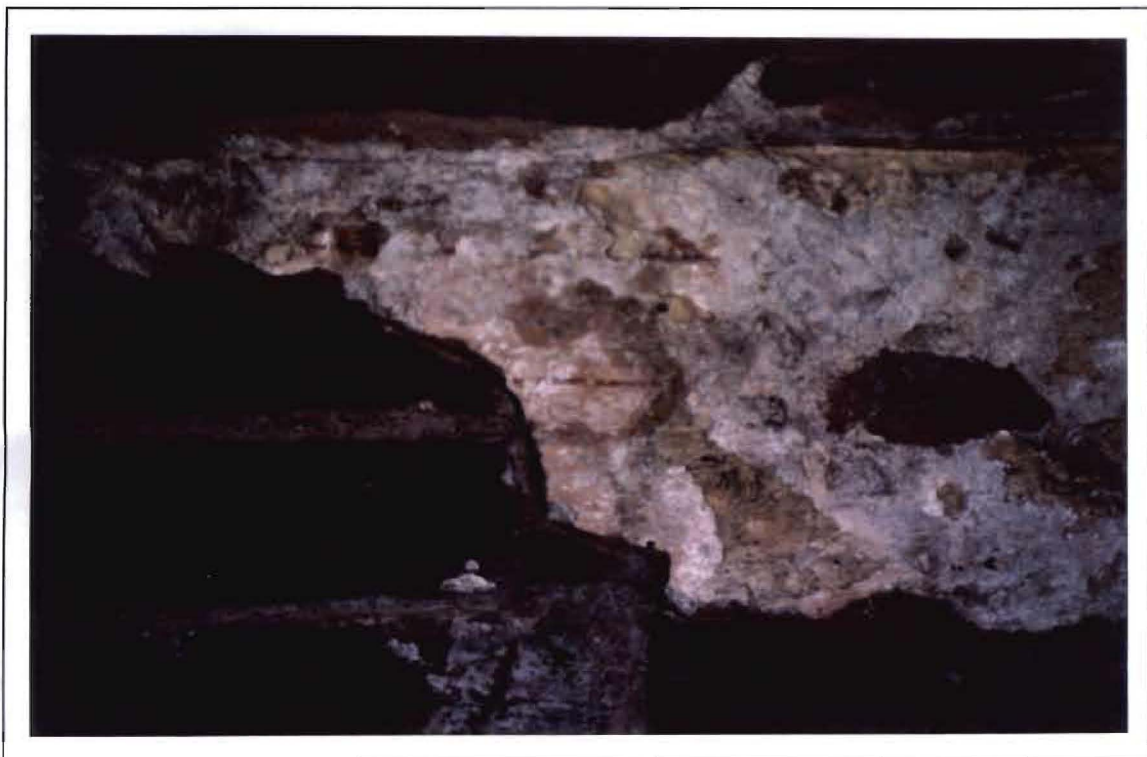
South wall, east window recess, soffit, remains of painted plaster
