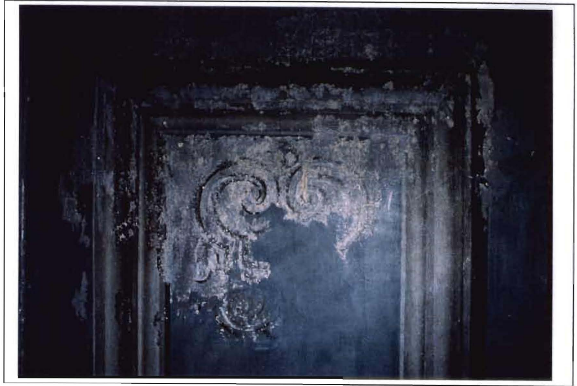
Northeast ante-room, north side, area uncovered in 1990
