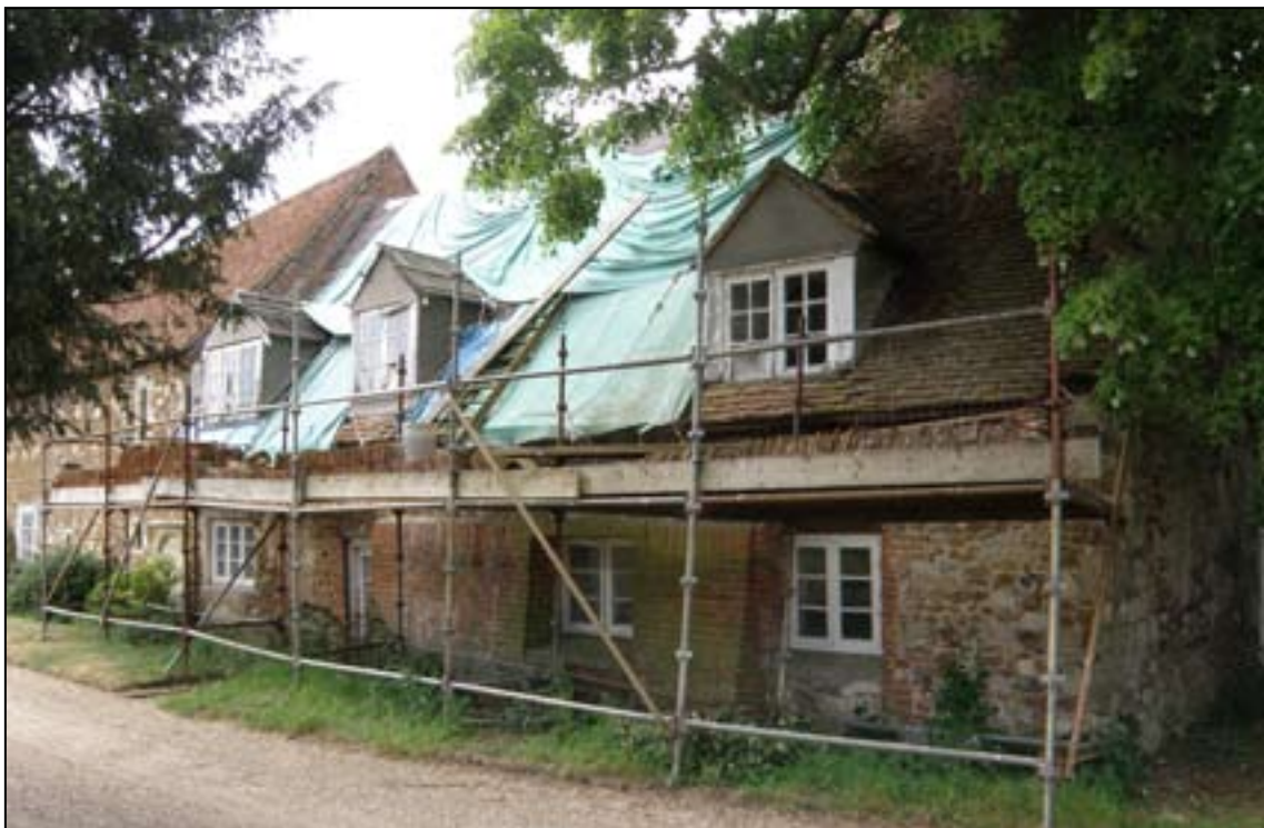
Fig. 13. The east front of the Bailiff's Cottage.
