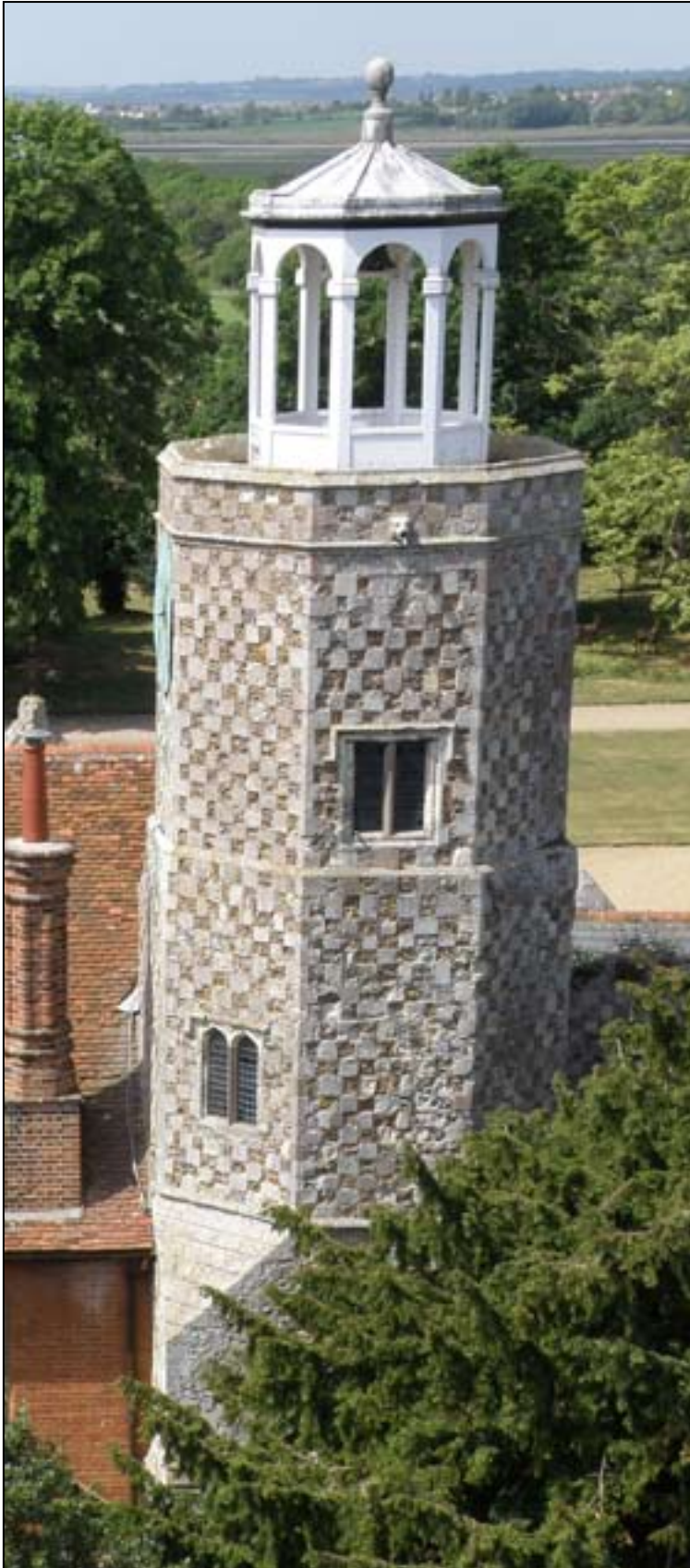
Fig. 26. The Clock Tower. © Pete Smith P5132866A.JPG
