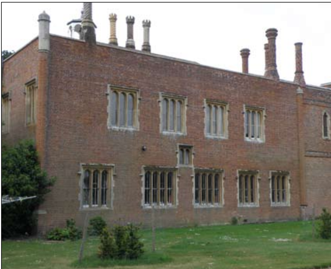
Fig. 23. The Service Wing built in the 1860s and altered internally in the 20th century. Pete Smith P5132850.JPG
