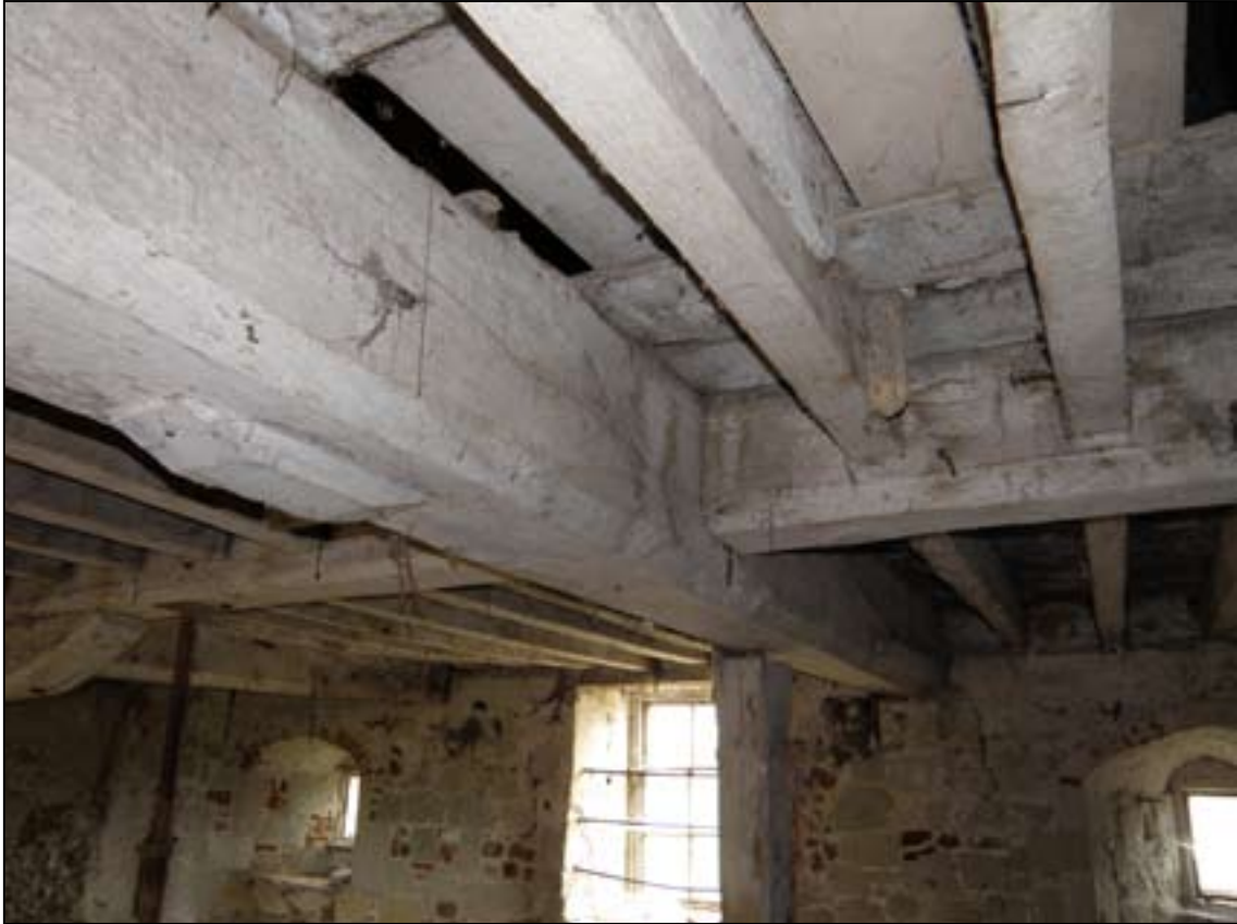
Fig. 12. The interior of the West Barn.
