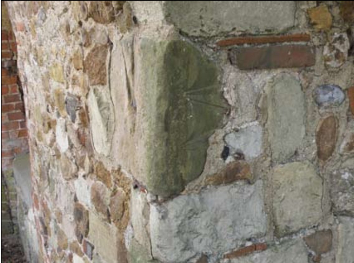
Fig. 14. A former medieval capital re-used as a corner stone to the Bailiff's Cottage. © Pete Smith P5132889.JPG
