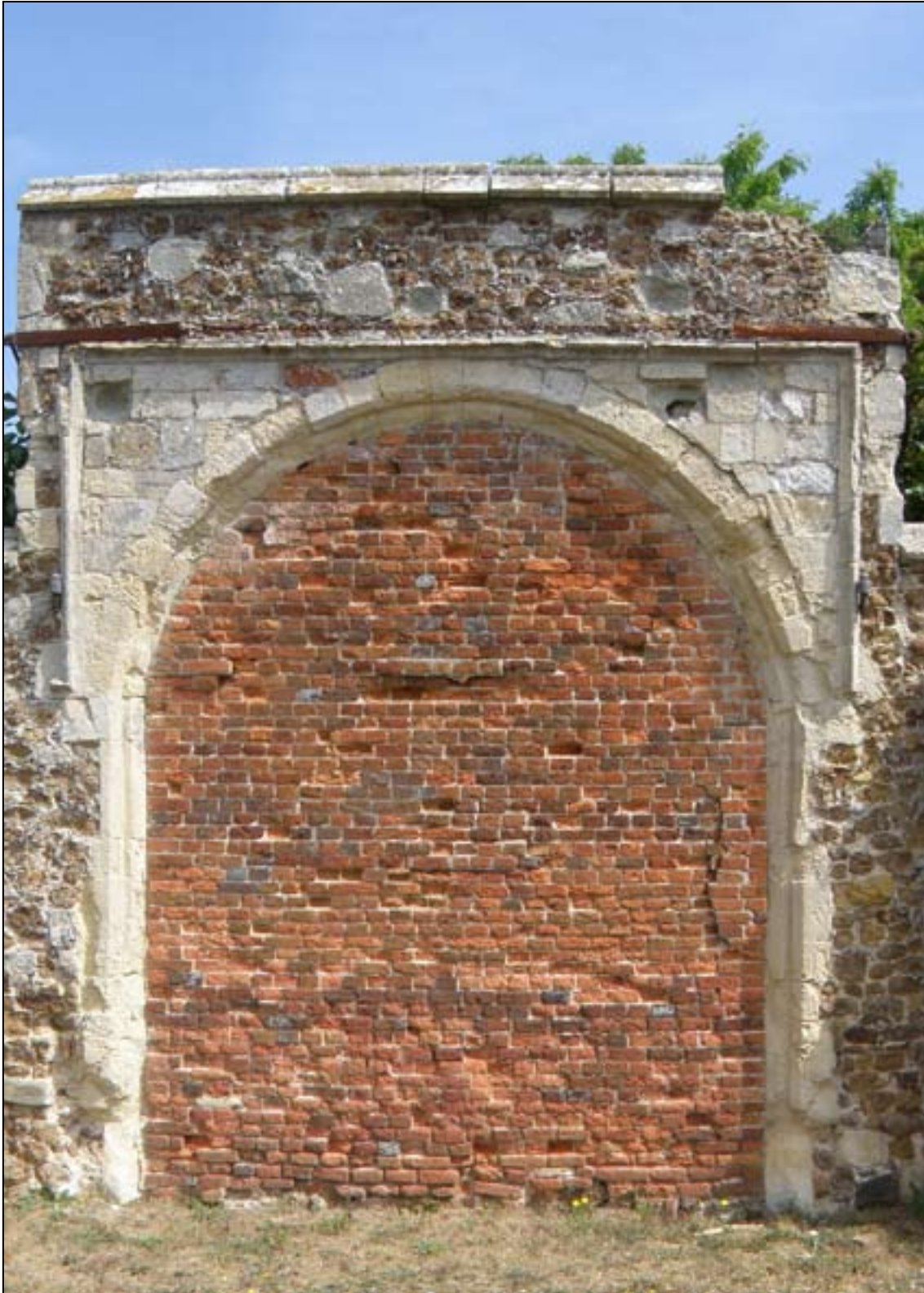
Fig. 39. The now blocked gateway inserted in the precinct wall as the main entrance to Lord Darcy's new house built in the mid-16th century.
