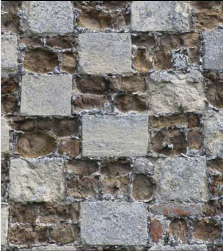
Fig. 30. A detail of the distinctive limestone and septaria chequerwork with flint galleting on the Abbot's Tower.
