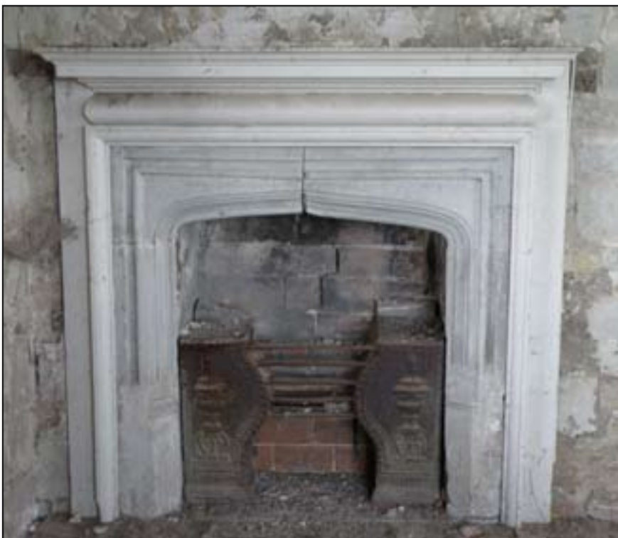
Fig. 31. A surviving 16th century fireplace with an added early 18th century fire surround, and a late 18th century basket grate in the Abbot's Tower.
