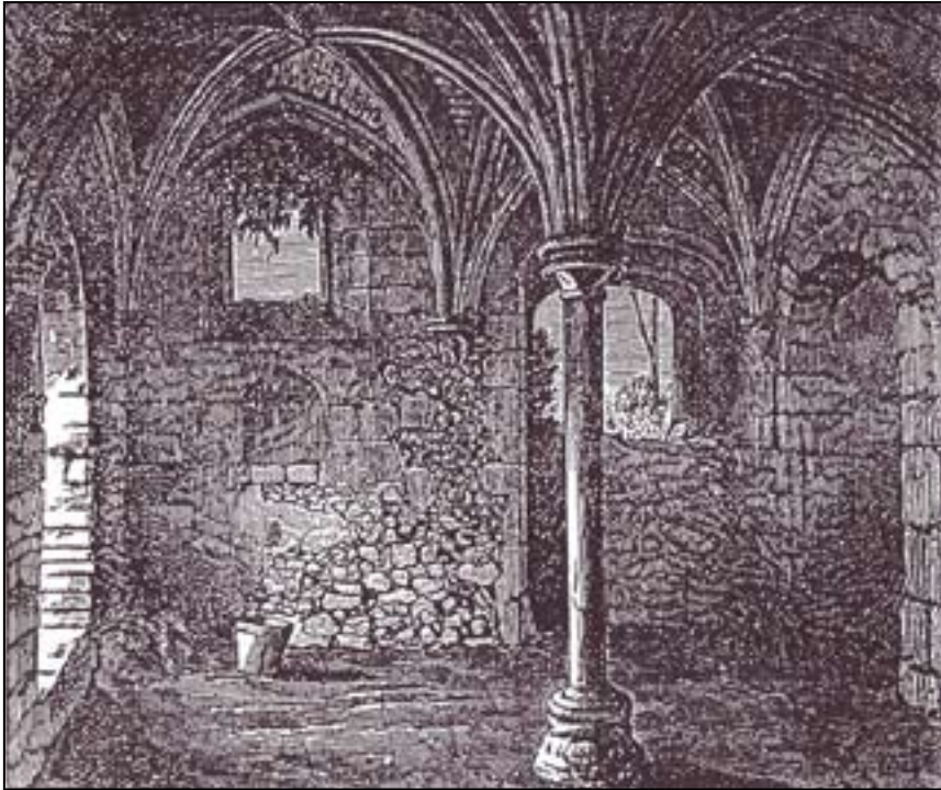
Fig. 34. An engraving published in 1873 showing the ruined former passage to the frater range of the monastic buildings before its conversion into the Chapel.
