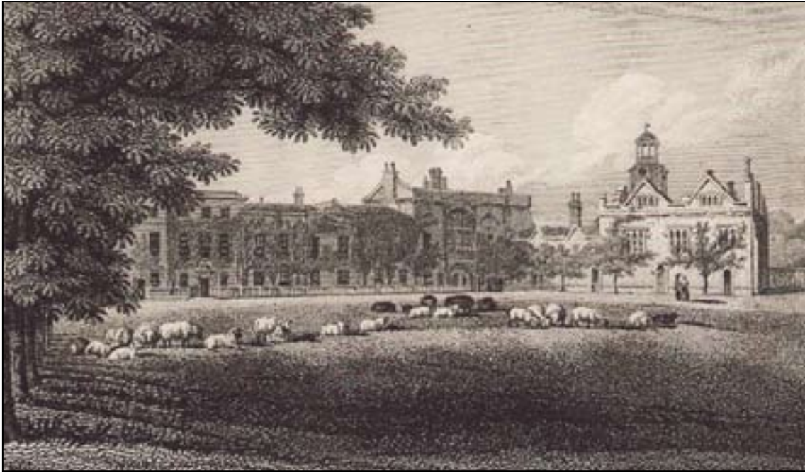
Fig. 15. An engraved view of St Osyth's Priory from the south-west, from Excursions Through Essex, 1819. The 18th Century House which was largely demolished in 1859 is partially visible on the left.
