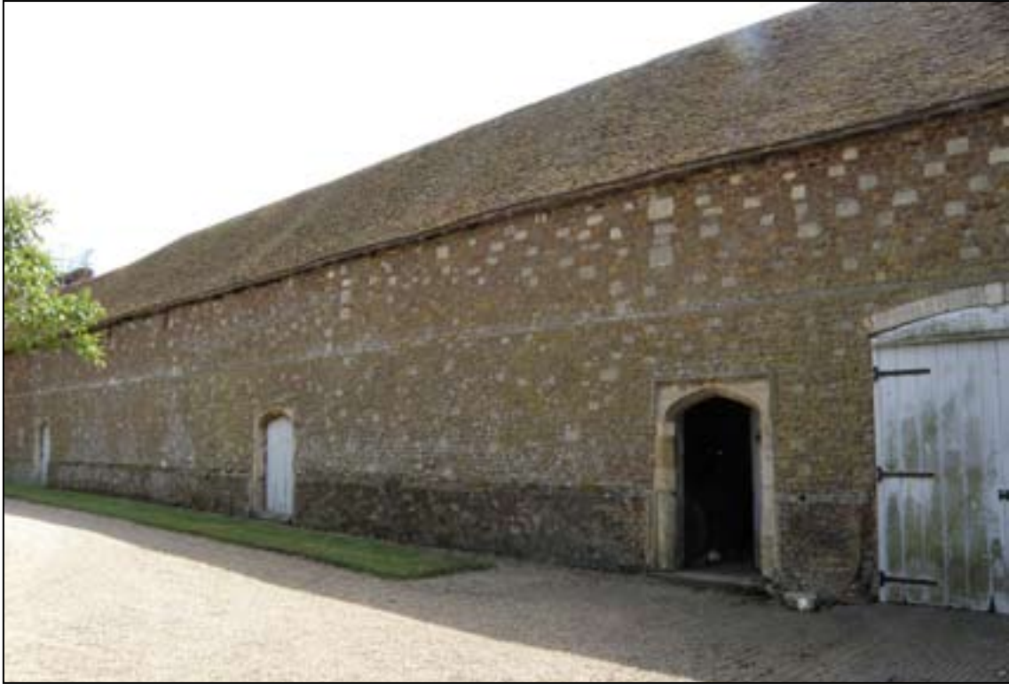
Fig. 4. The north stone wall of the Tithe Barn.
