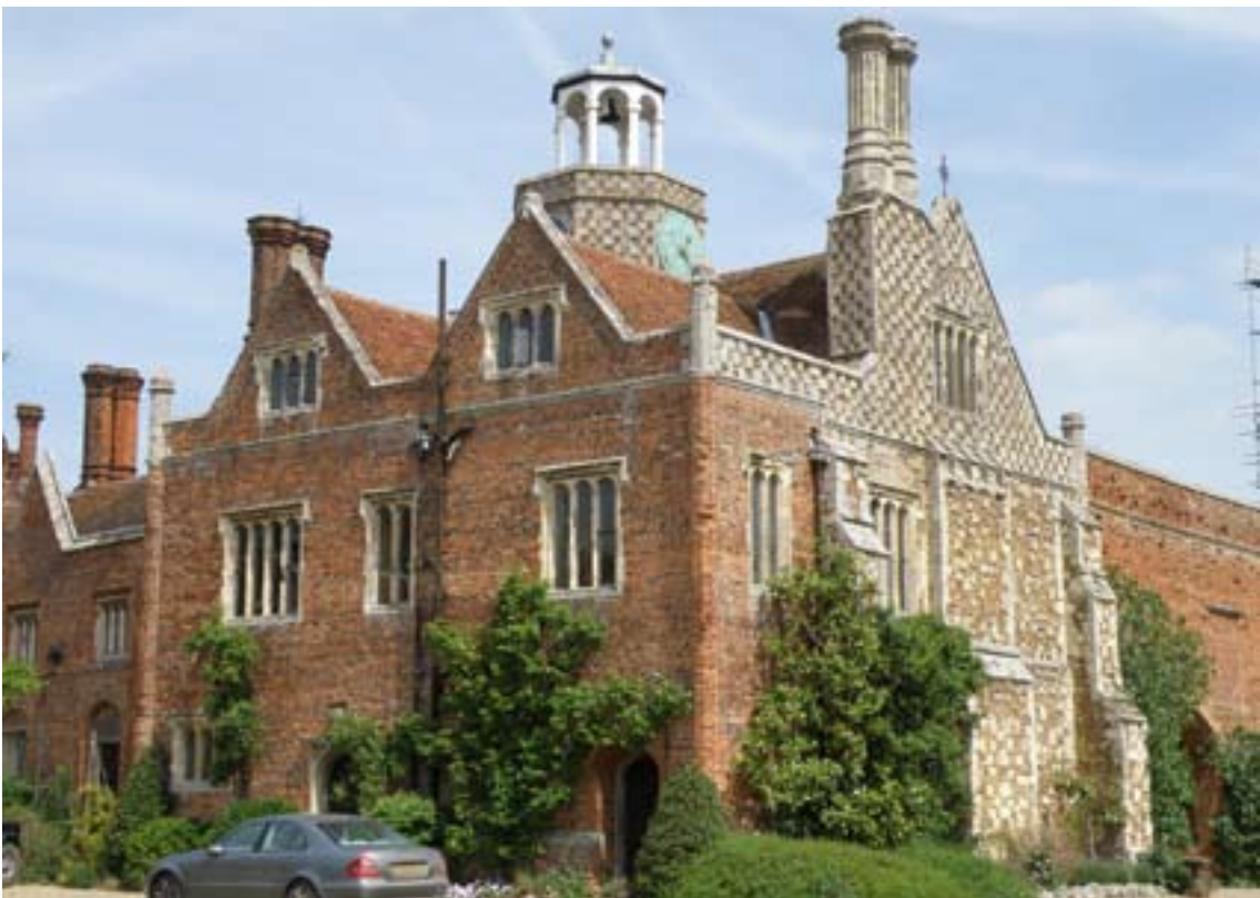
Fig. 25 The south and east fronts of the South Wing. © Pete Smith P5132913.JPG
