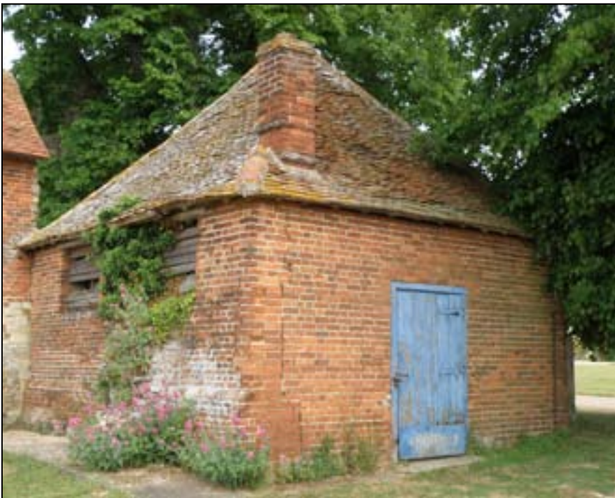
Fig. 10. The Drying House.
