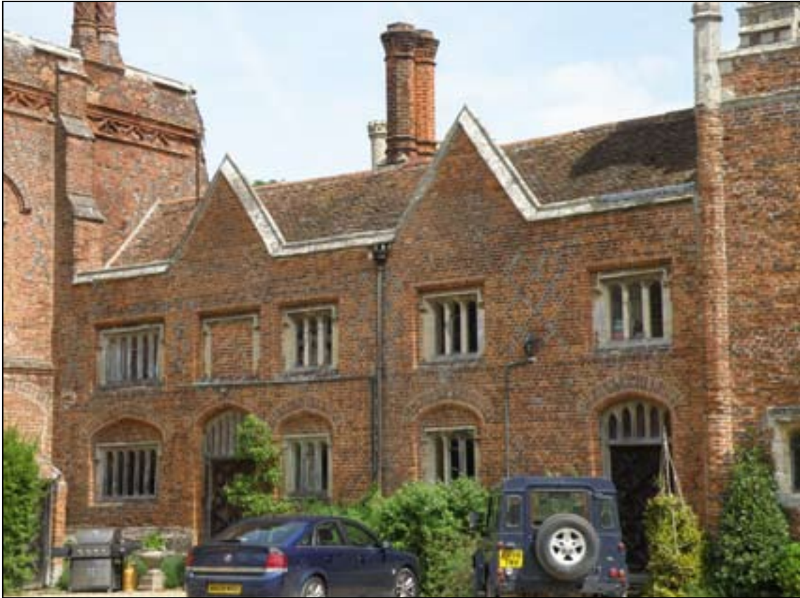
Fig. 24 The northern section of the east front of the South Wing. © Pete Smith P5132912.JPG
