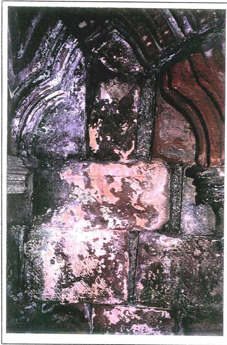
Vestibule into Chapter House, northwest blind arcade, north side
