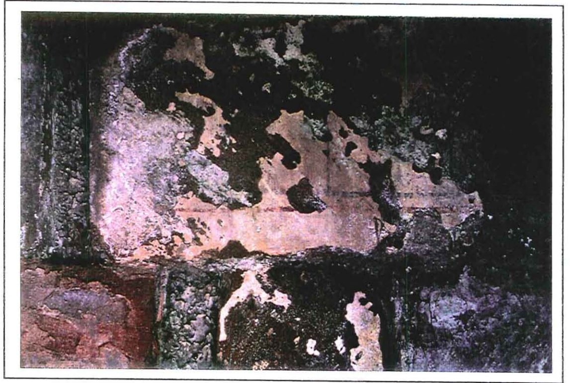
Detail, masonry pattern within northwest blind arcade
