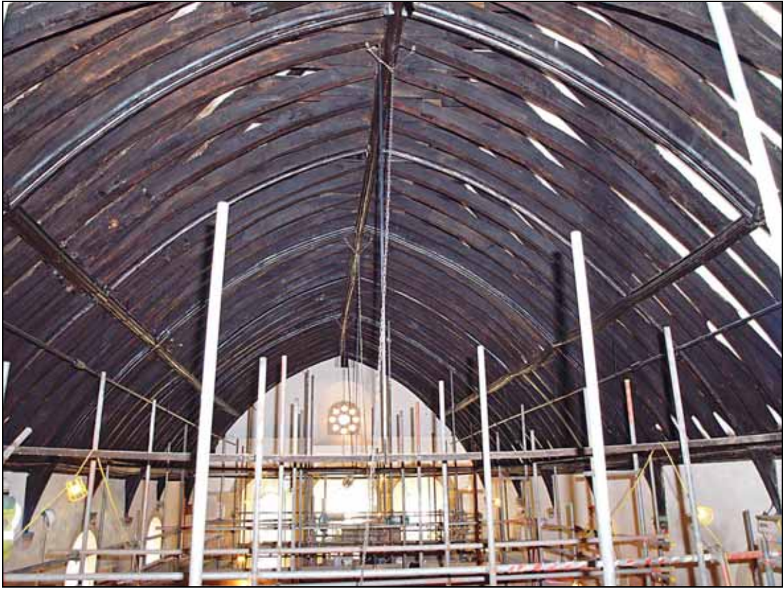
Figure 6: Nave roof (Keystone Historic Buildings Consultants)
