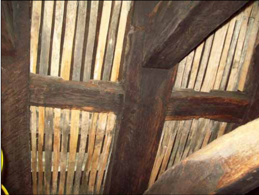
Figure 5: The false 'purlins' of the chancel roof
