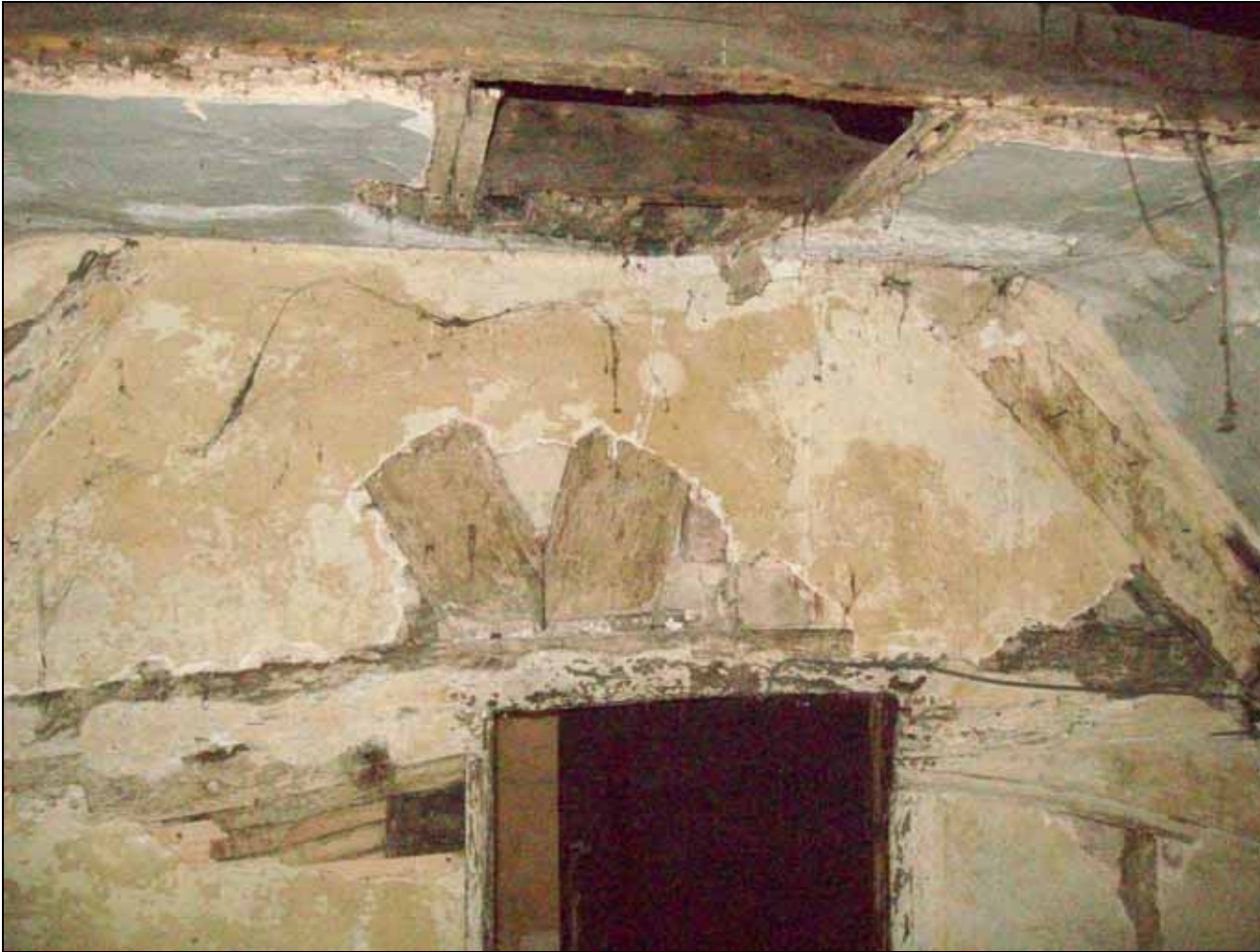
Figure 5: Central truss (south face)
