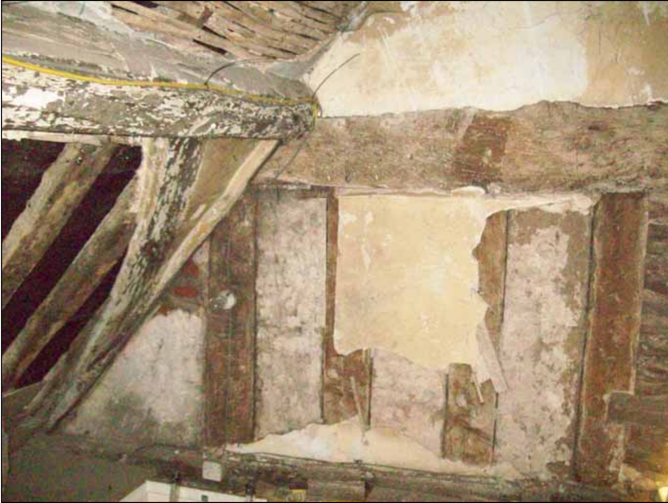
Figure 4: South gable truss (north face)
