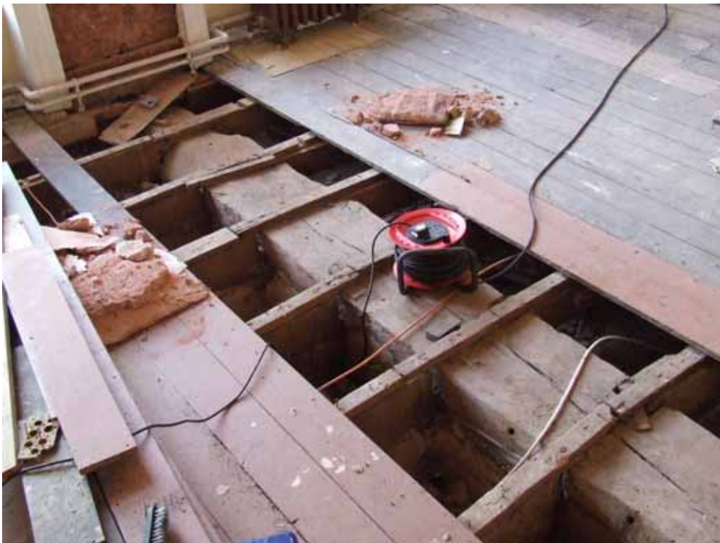
Figure 4. View of one of the beams exposed during recent works
