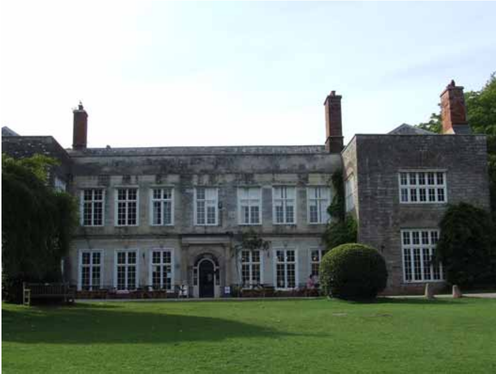
Figure 3. External view of the house from the south-west, looking north-east
