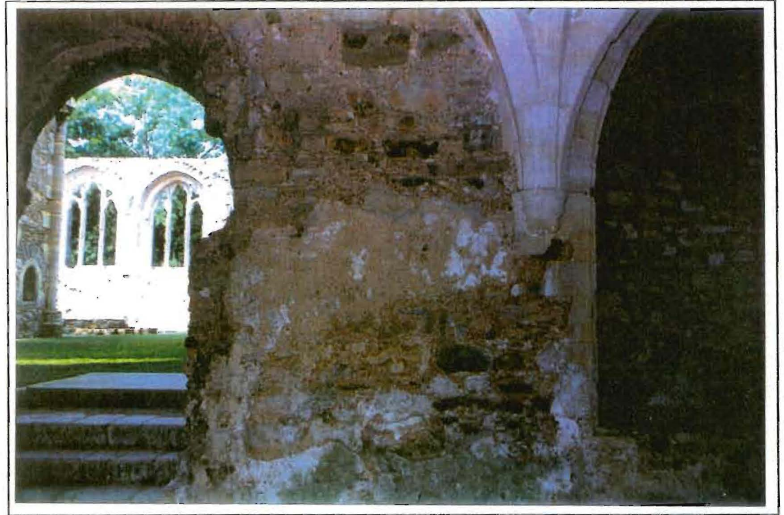
Chapel, north wall, area of plaster with faint traces of paint
