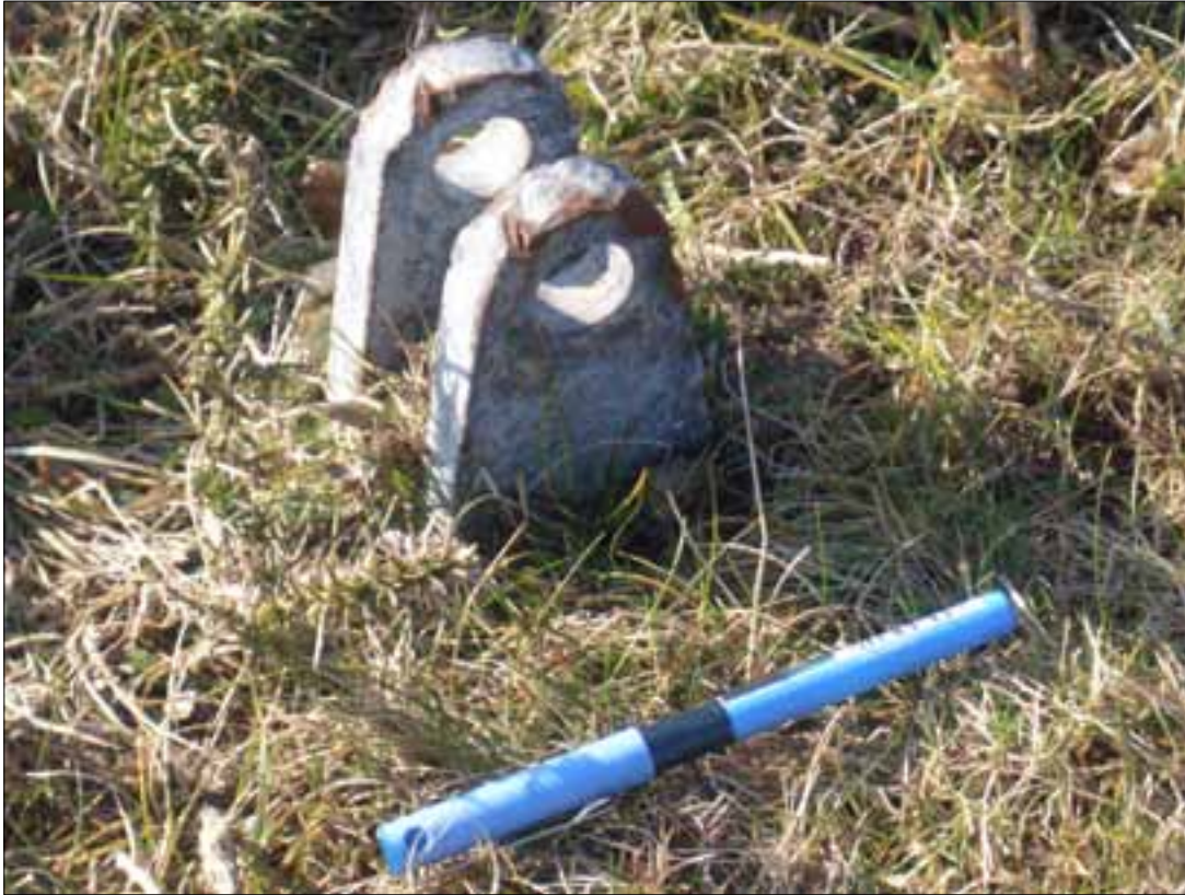
PI 7: Central bracket interpreted as the step for a collapsible mast on the Garrison, possibly of Second World War date, 2010.
