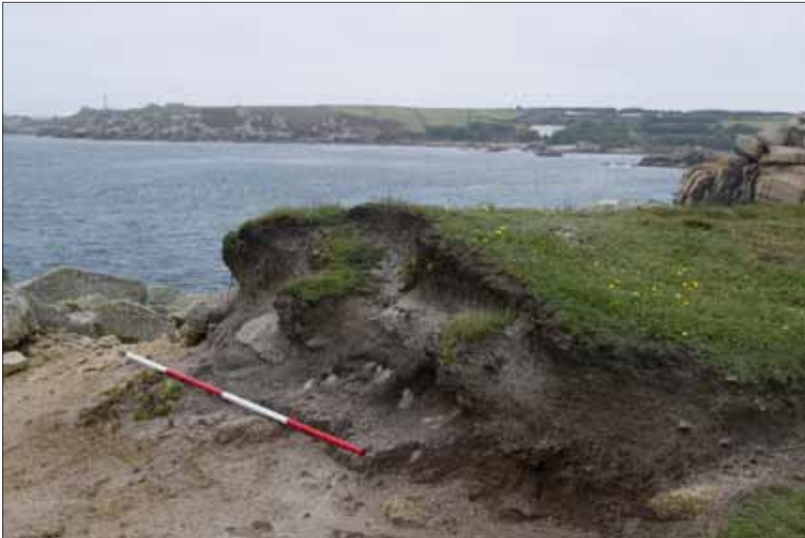
Pl 10: Eroding section of the supposed battery rampart at Church Point, St Mary's, 2008.
