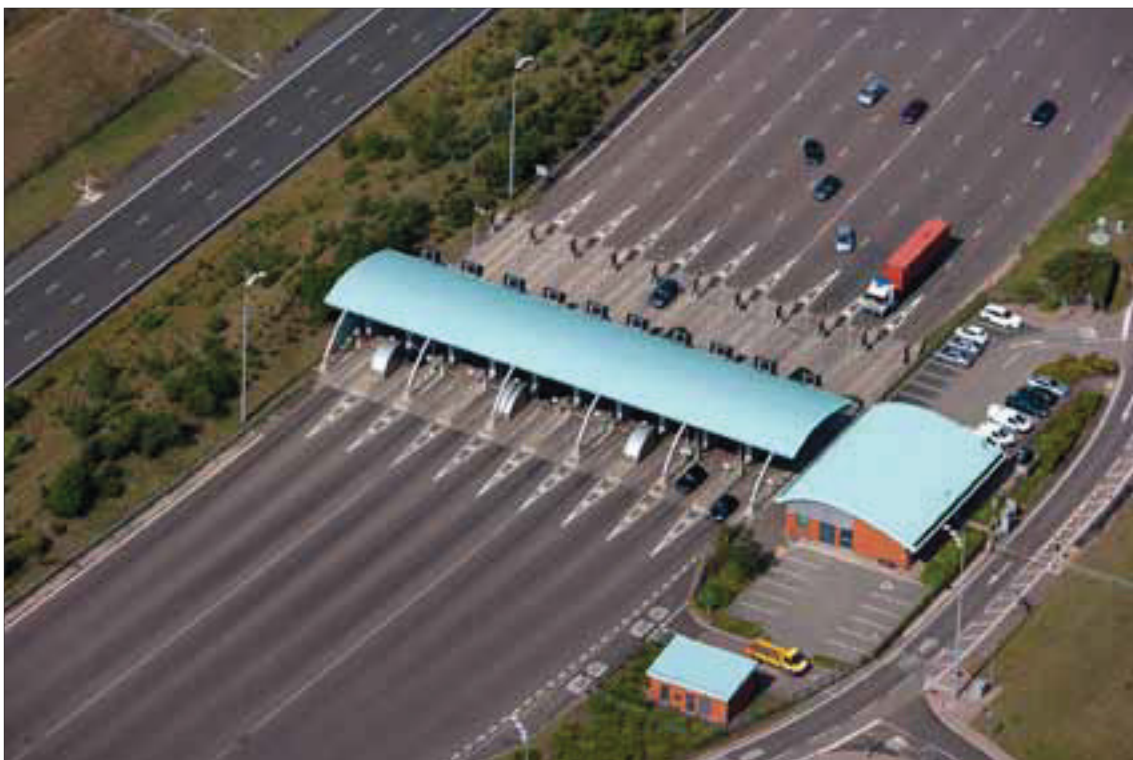
Figure 9 - Toll booths on the M6 Toll (© English Heritage.NMR 26738/035)
