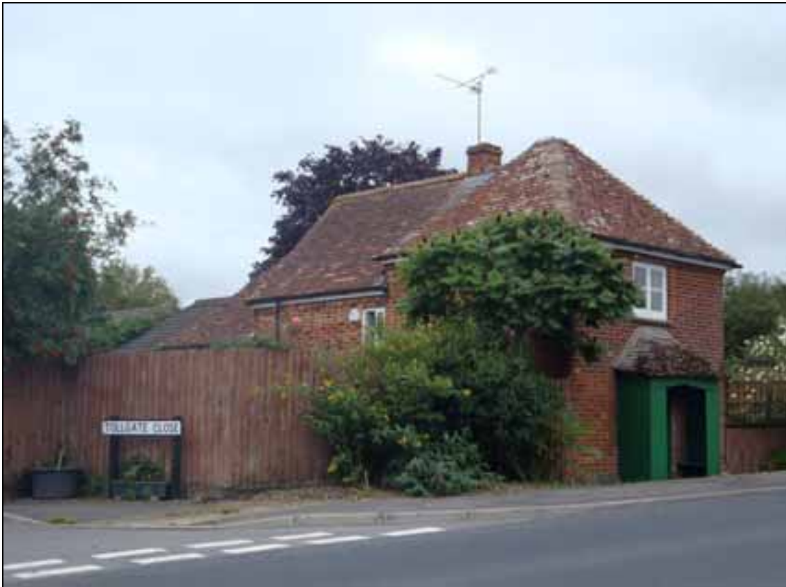
Fig 7: Amesbury Countess toll house. The toll house has given its name to the recent cul-de-sac immediately to its south-west.
