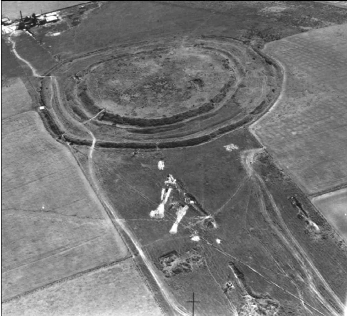
Fig 11: Castle an Dinas mine in production. The aerial photograph shows the adits to the north of the hill in the foreground and the alignment of blondin pylons extending over the hill towards the southern shaft. Extract from HV56 taken 24th June 1952: original photography held at Cambridge University Collection of Aerial Photography.
