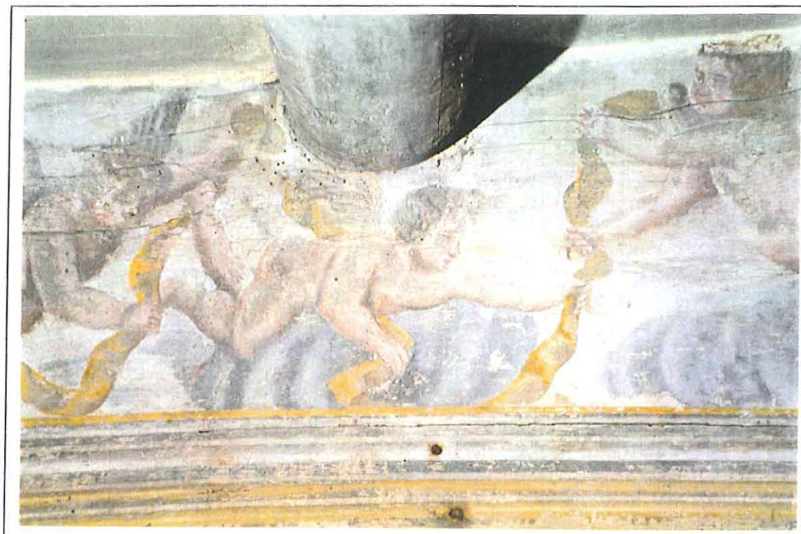
St Anne's Chapel, detail of painted beams
