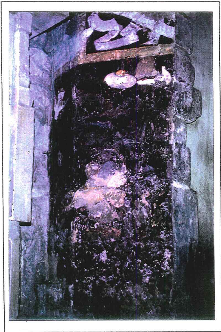
East range, east wall, south window, south splay
