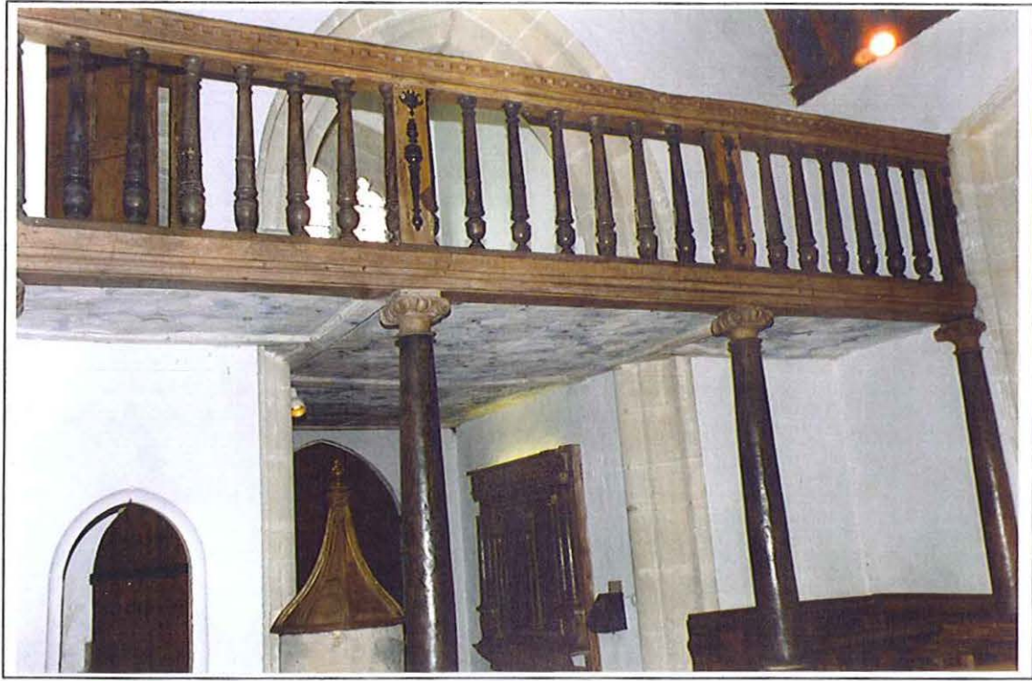
Western Gallery, general view to west
