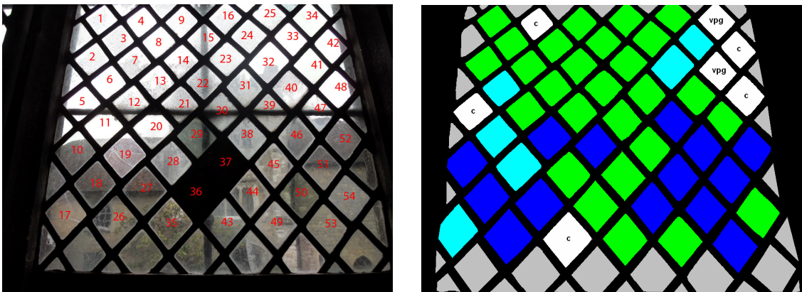
Figure 19 W02 Panel 2 showing the spatial distribution of glass types (see Figure 18 caption)
