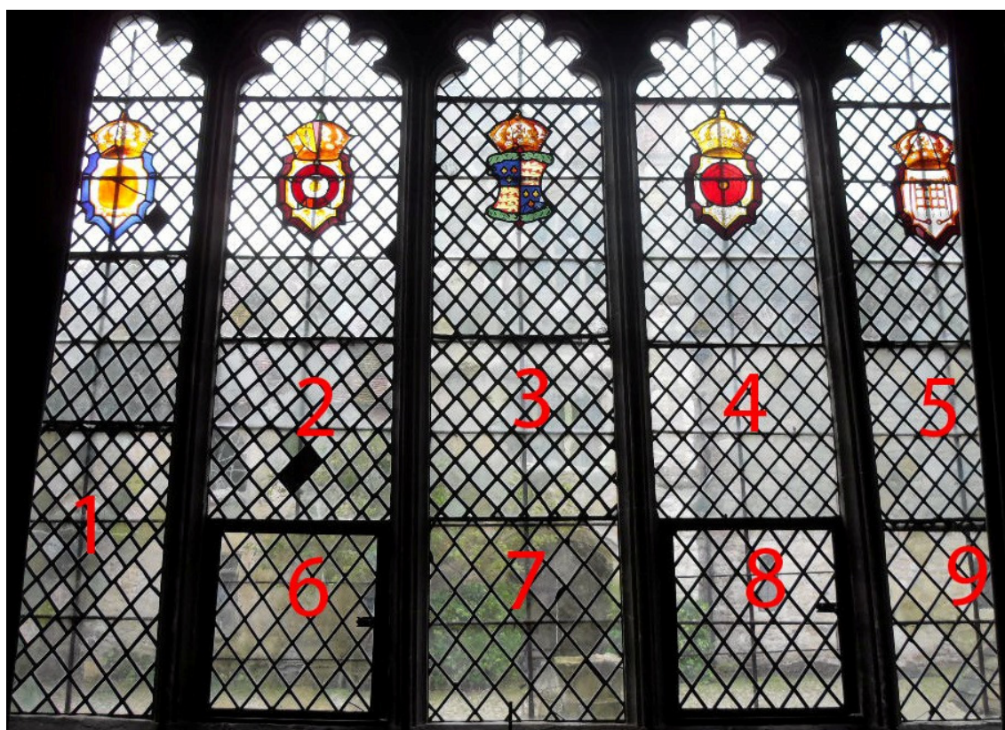
Figure 14. W02 showing the location of the analysed panels (note the different sizes of pane in Panel 1)
