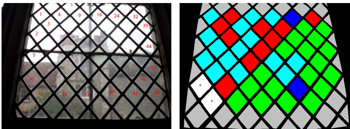
Figure 21 W02 Panel 4 showing the spatial distribution of glass types (see Figure 18 caption)
