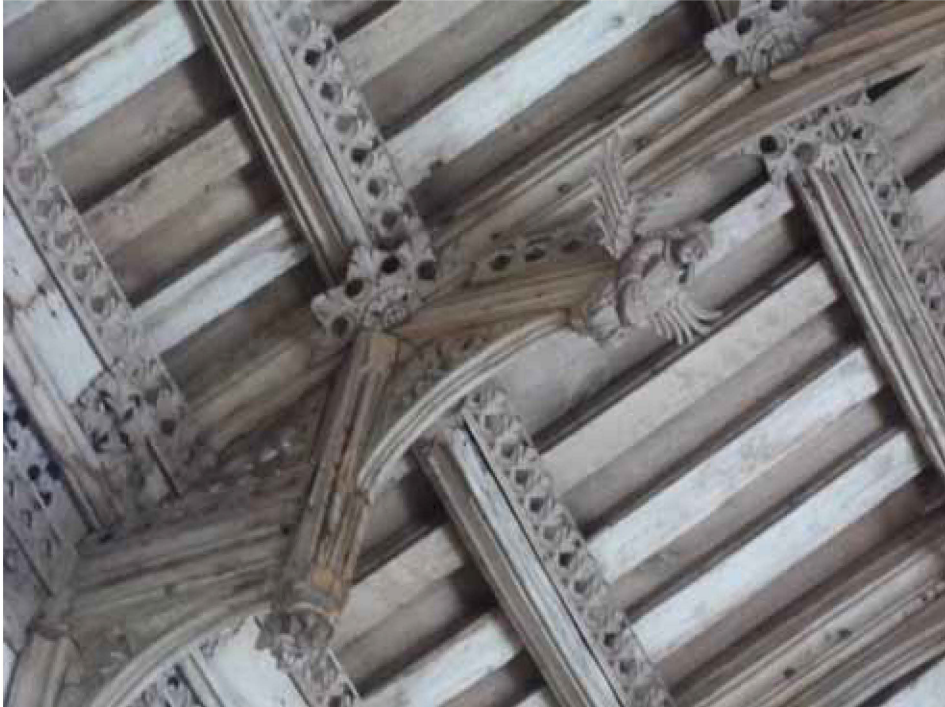
Figure 3b: Detail of a hammer beam truss
