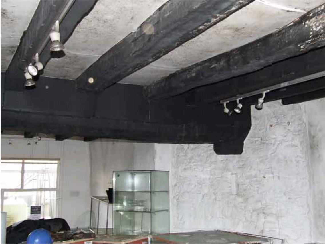
Figure 8. View of the north-south beam (centre of photograph) sampled as dtm 16
