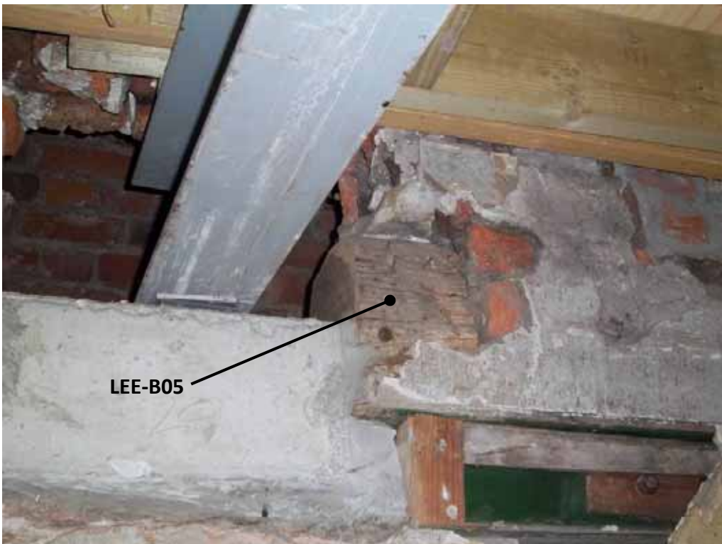
Figure 3a/b: View of the framing to the north wall (top) and the single horizontal timber of the south wall (bottom), cut off to allow for the insertion of the steel joist, sampled as LEE-B05
